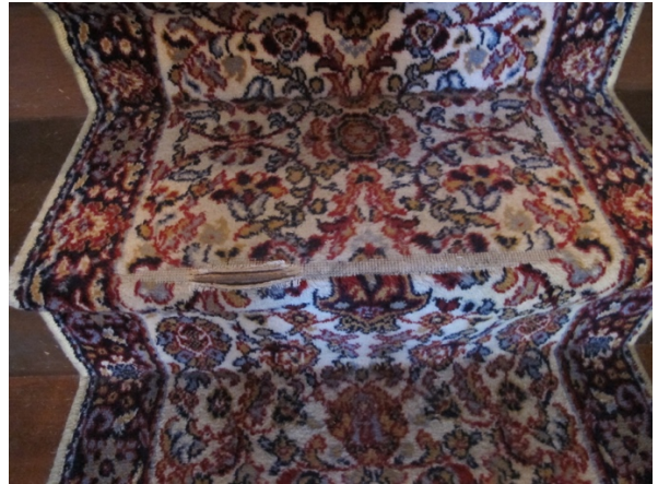
Wear and tear at the edge of the stair runner from foot traffic. The gap in the weave is a trip hazard.
