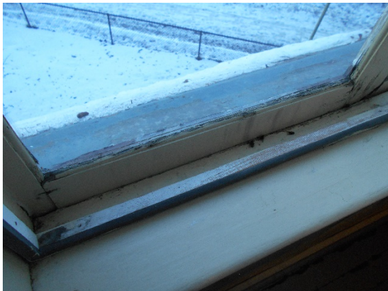
Deteriorated sash (December, 2017) (repair, reseal, and repaint)
