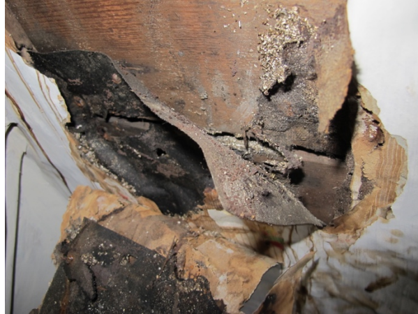
Detail of exposed roof elements revealed by the water damage.
