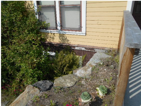
Peeling Paint – south basement
