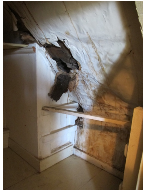
Interior of boys' room cubby with significant water damage in the eastern wall.
