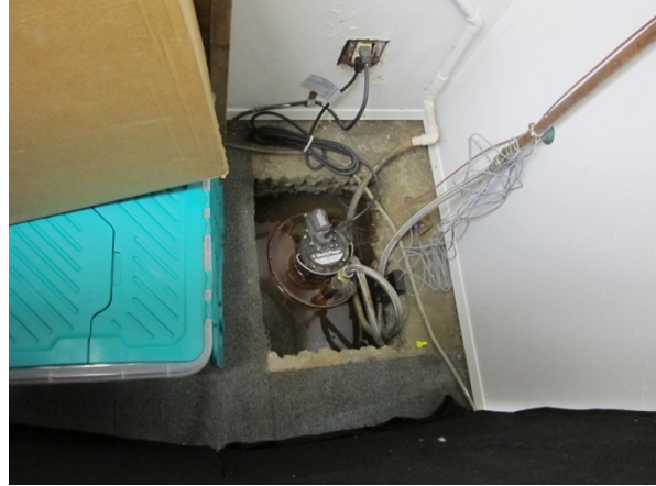
Exposed sump pump with standing water in the southeast corner of the basement conference room.
