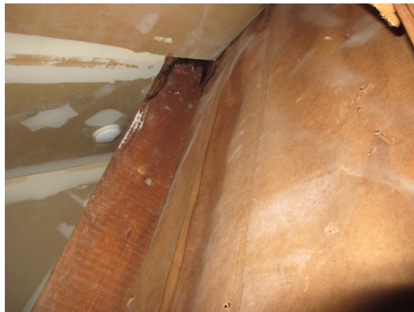
West wall of girl's room cubby with water damage.
