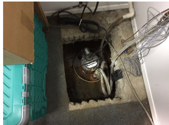
Open Sump- Basement Conference Room (remove when site drainage repaired)
