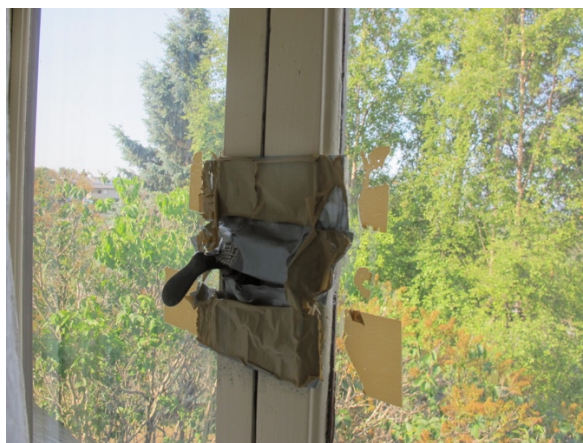
Broken window that has been duct taped shut.
