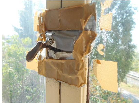
“Bandaged” casement operator (repair & refinish windows & hardware)
