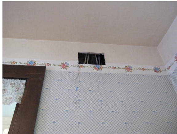
Cutout hole in the north wall of the kitchen that allows access to wiring.
