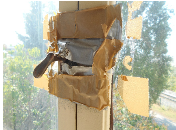
Damaged Window Hardware- dormer
