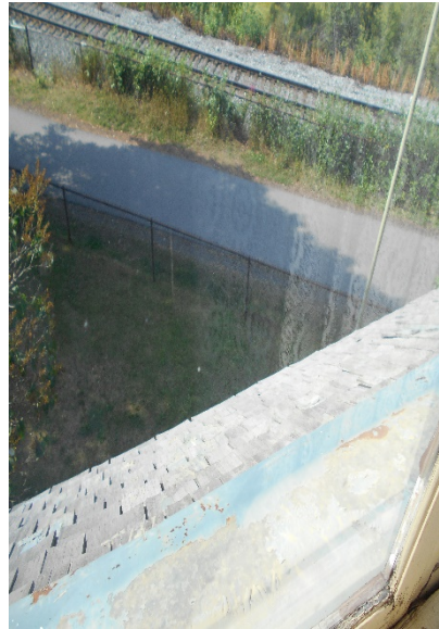
West Dormer Shingles (faded, broken shingles)
