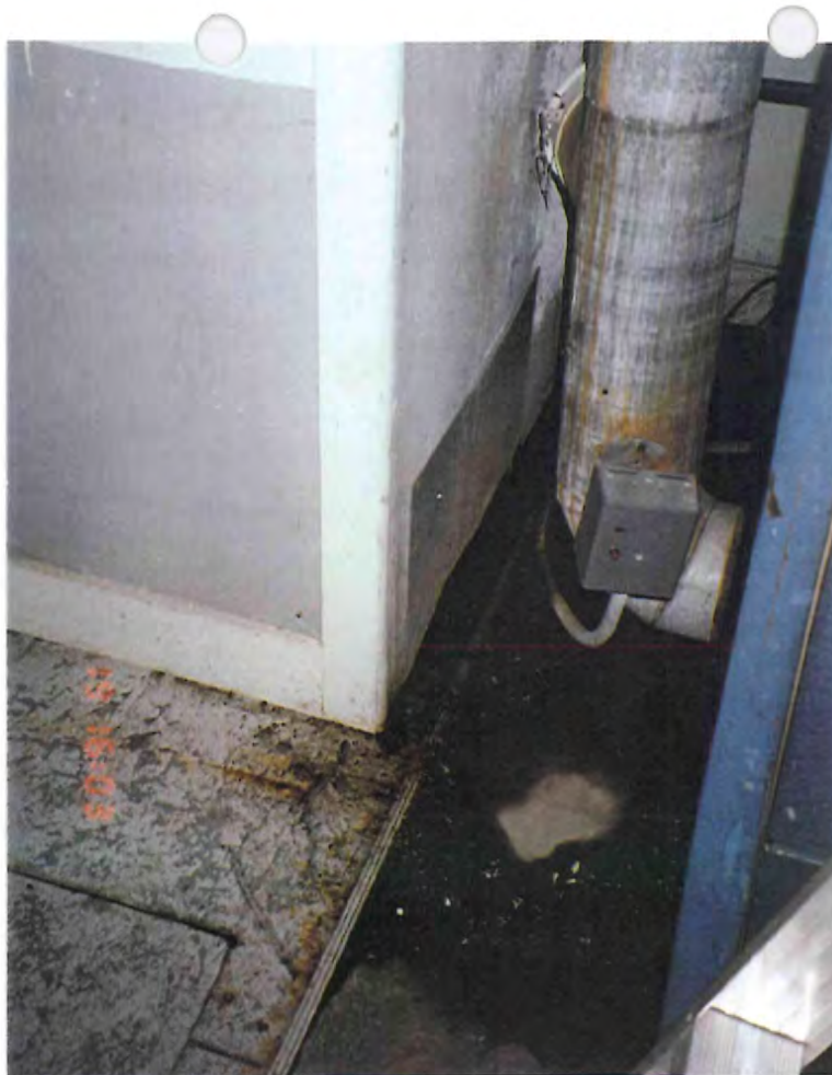
Plate 5 Cement asbestos board behind and below furnace in Building 2. Note rust stains on flooring and wet stains due to water leakage around furnace chimney.
