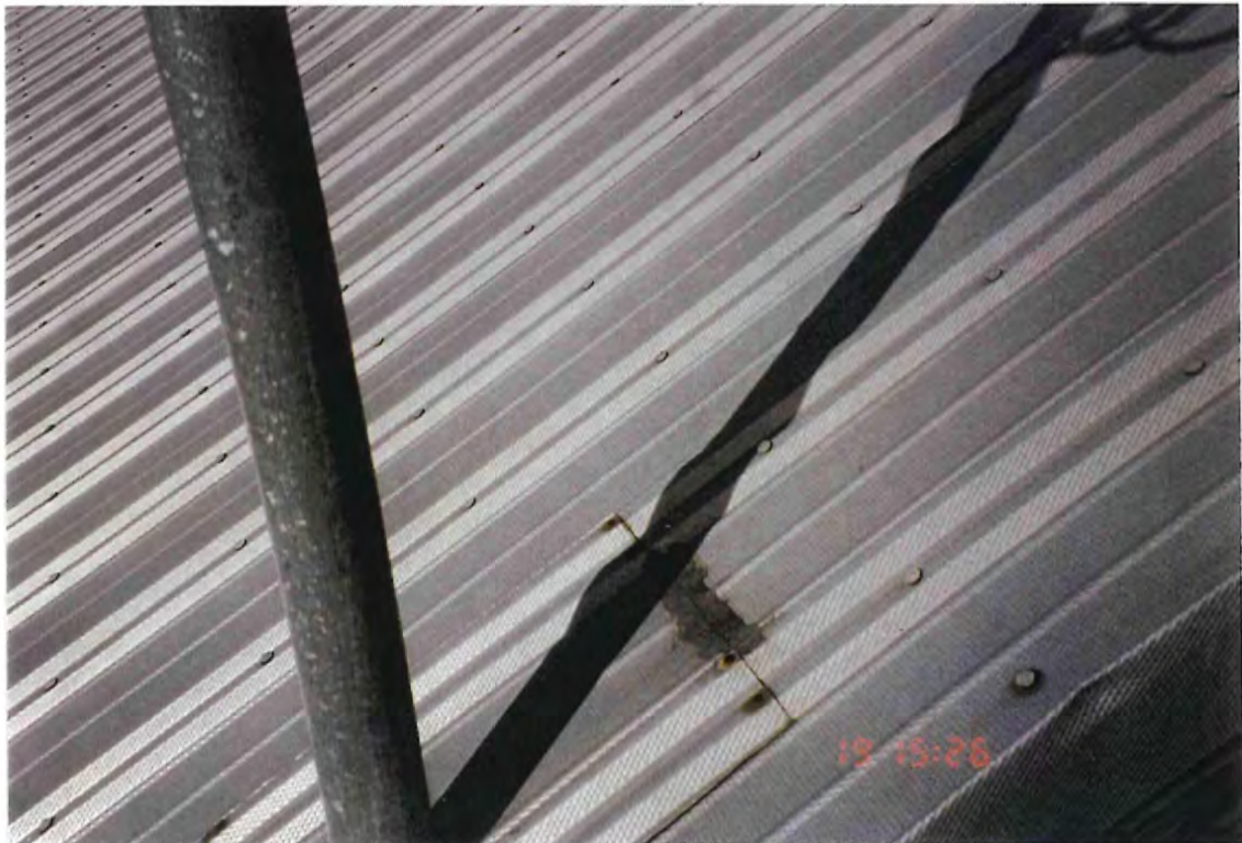
Plate 4 Asbestos-containing gray fibrous patching on aluminum roofing of Building 1.
