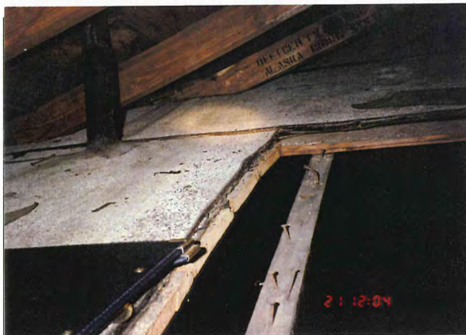
Plate 14 Asbestos-containing grit surfaced roofing of original section of Building 3. Note lead flashing on plumbing vent pipe and "new" rafters laid on "old" roofing.
