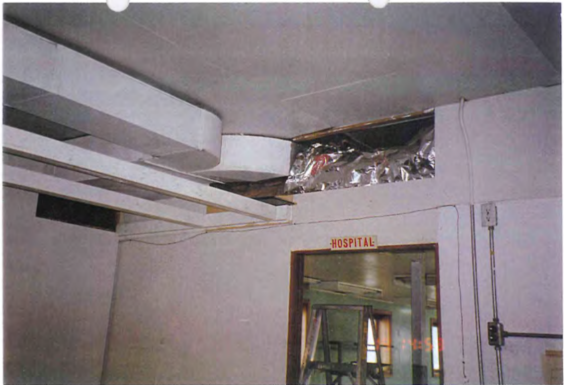
Plate 1 Looking south in north room of Building 1. Gypsum wall board walls and ceiling without joint compound. Note ducts exposed with lead seal at seams, and concealed ducts in south room. South room has gypsum wall board walls and ceiling with asbestos-containing joint compound, and fluorescent light fixtures with PCB Ballasts.
