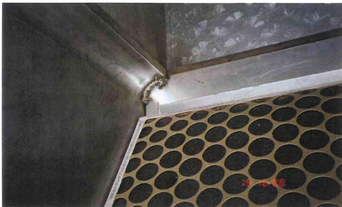
Plate 6 Asbestos-containing gasket in return air plenum of furnace in Building 2.
