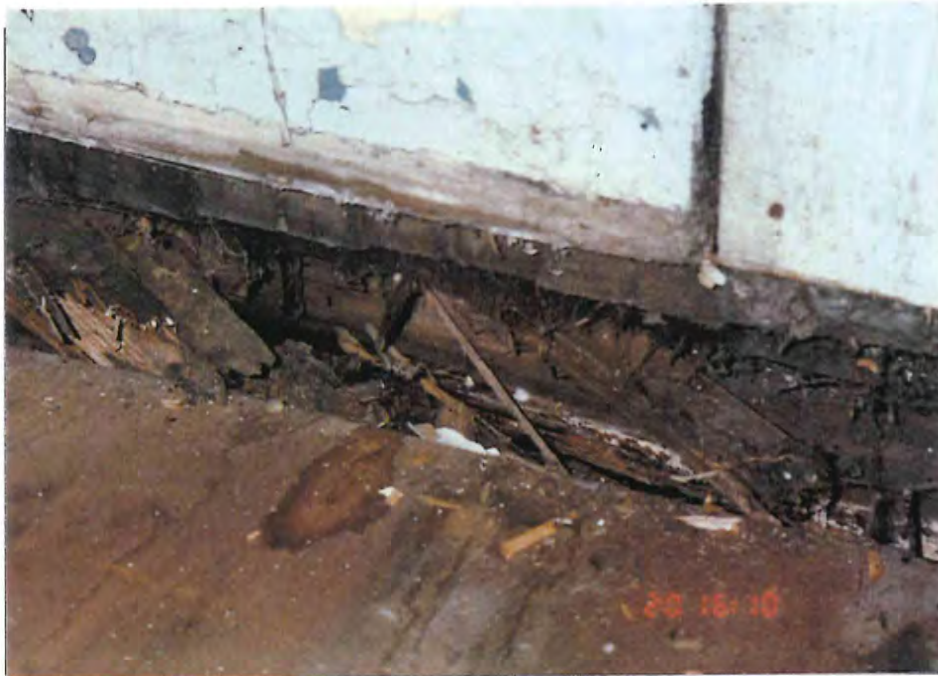
Plate 11 Exterior wall, west central room of Building 3. Note floor dropped 4 inches, exposing horse hair and tar paper between layers of wood. Note dry rot.
