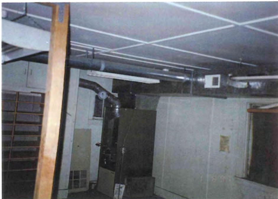
Plate 9 South room of Building 3. Note furnace with attached gas line and abandoned oil piping and filter. Note fluorescent lights with PCB-containing ballasts and shelved cabinet with cement asbestos board lining.
