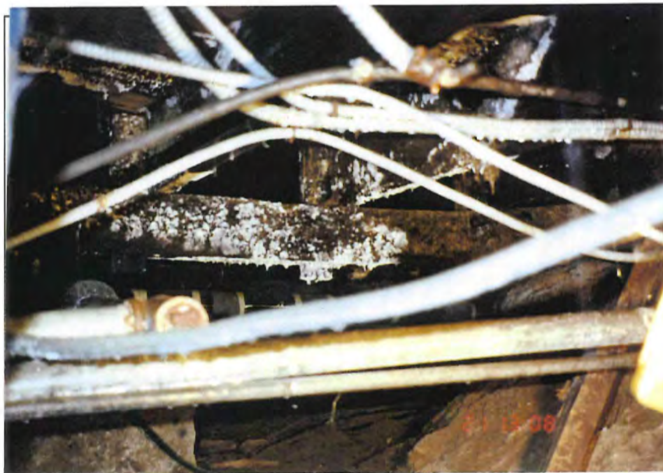
Plate 12 Crawl space from access hatch at stairs to basement, Building 3. Note moisture drops and fungal growth on wood structure.
