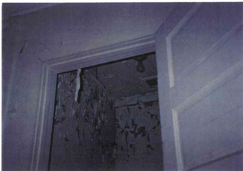
Plate 10 Peeling paint in bathroom of Building 3.
