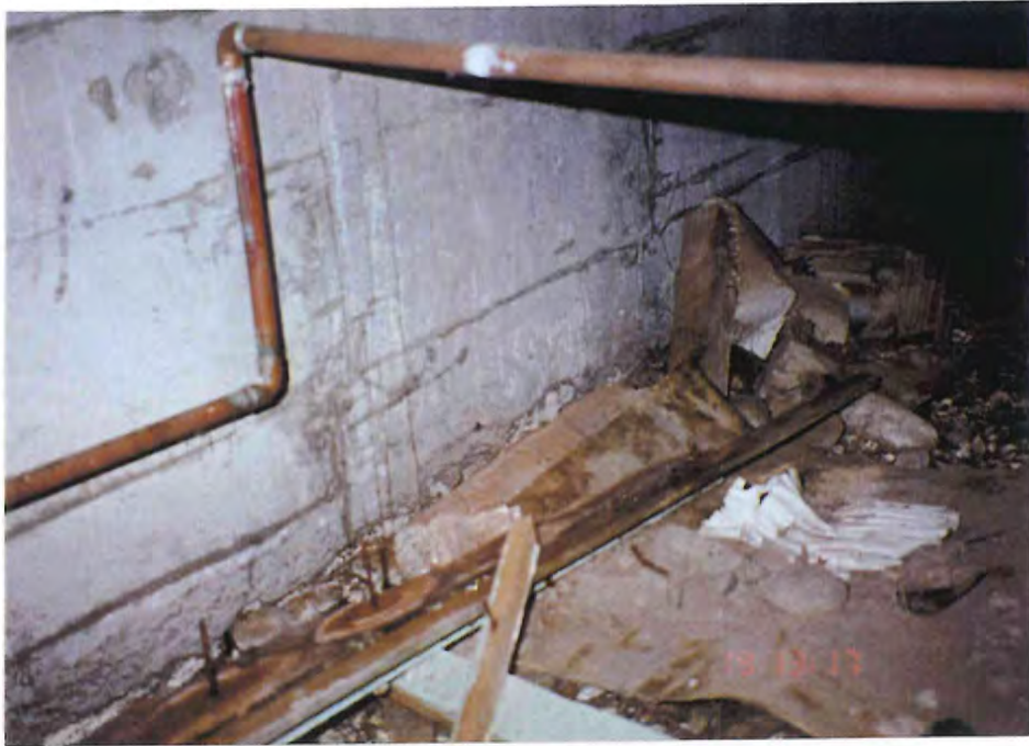
Plate 3 White asbestos-containing pipe insulation debris under central crawl space of west wing of Building 1. Note copper pipe replaced insulated steel pipe.
