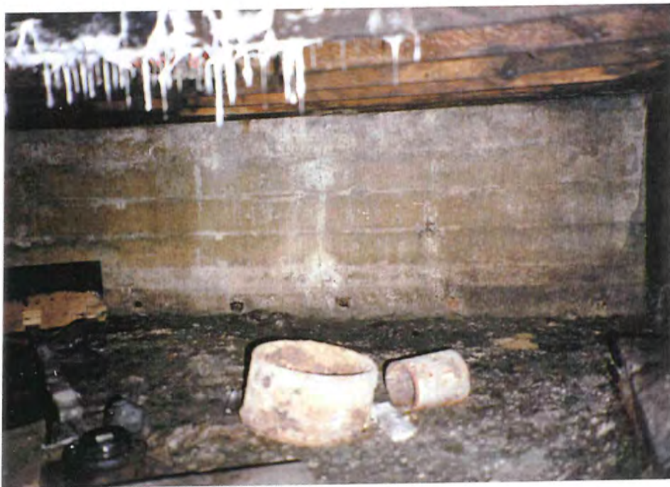
Plate 2 Note debris and fungal growth in crawl space of west wing of Building 1.
