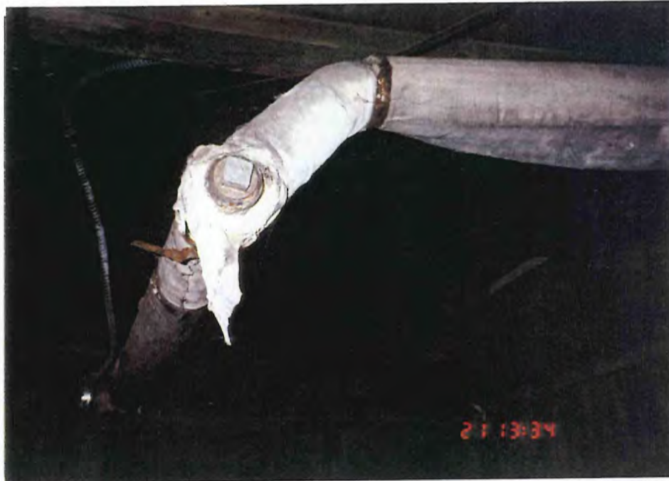
Plate 13 Damaged white asbestos-containing pipe insulation in basement of Building 3.
