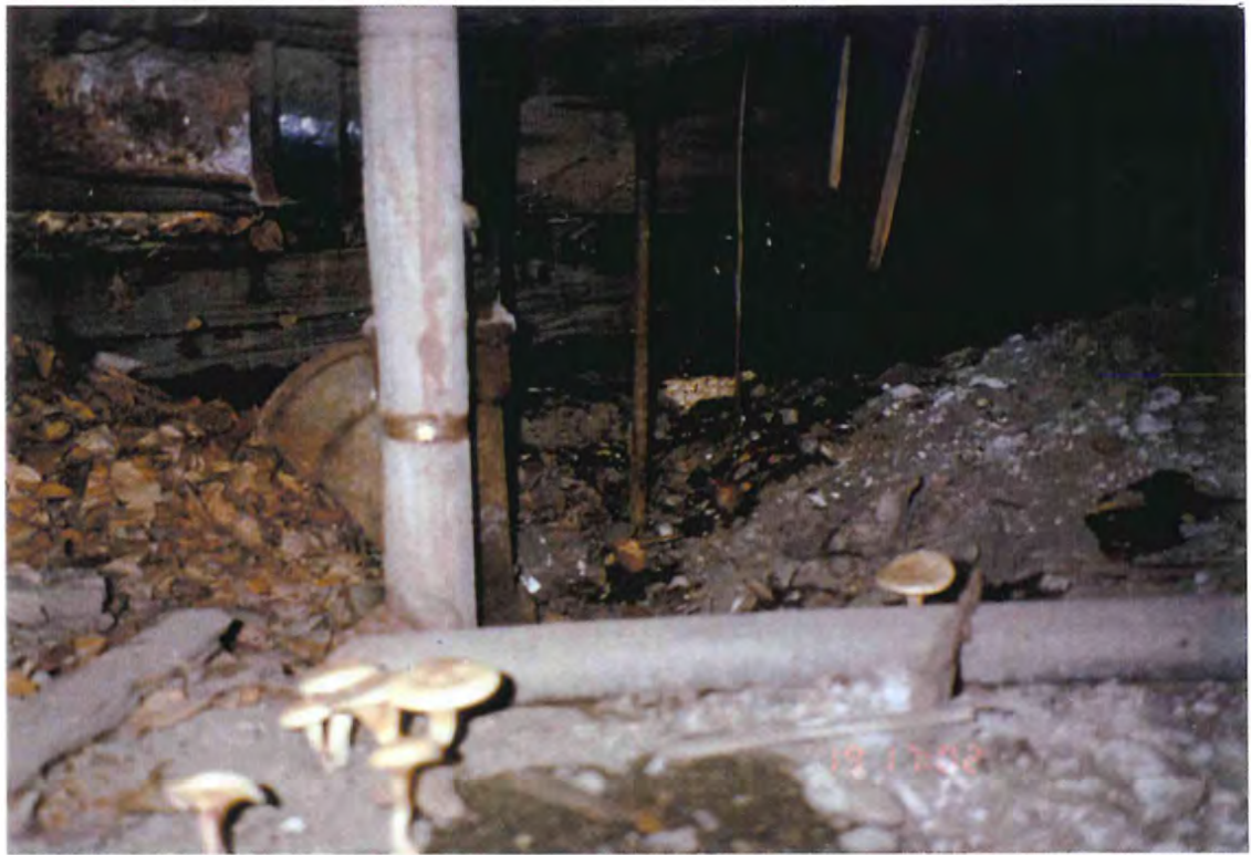
Plate 7 White asbestos-containing pipe insulation in crawl space of Building 2. Note wet floor beams, leaves blown into crawl space through wood skirting, and fungal growth.
