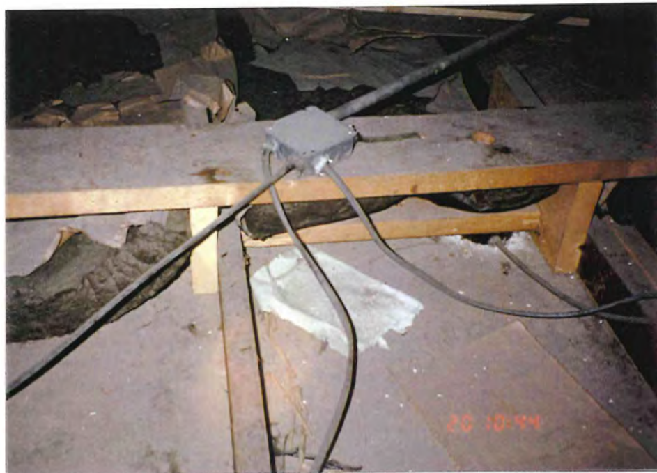
Plate 8 Asbestos-containing white paper in attic of Building 2.
