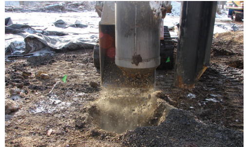
Vertical ramming to compact into thin lifts
