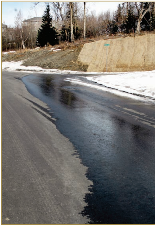
Cutbacks on road edges increase runoff on the road and adjacent property (above). Glaciation is a problem on some Hillside roads.
