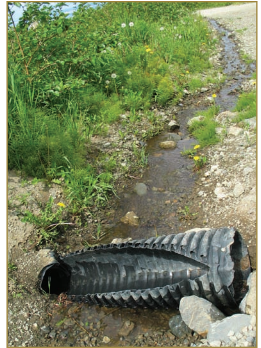
Evidence of the challenges of maintaining drainage infrastructure: culvert and drainage ditch along Clark's Road.
