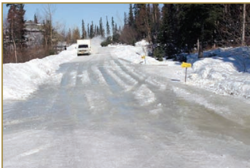
Cutbacks on road edges increase runoff on the road and adjacent property (above). Glaciation is a problem on some Hillside roads.
