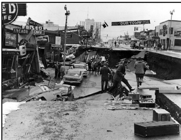
Graben formation on 4 th Avenue near C Street, Anchorage, 1964 Alaska Earthquake
