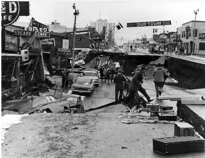
Photo 1.1 Collapse of Fourth Avenue near C Street, due to earthquake caused landslide. Before the earthquake, the sidewalk at left, which is in the graben, was at street level on the right. The graben subsided 11 feet in response to 14 feet of horizontal movement. Source USGS.
