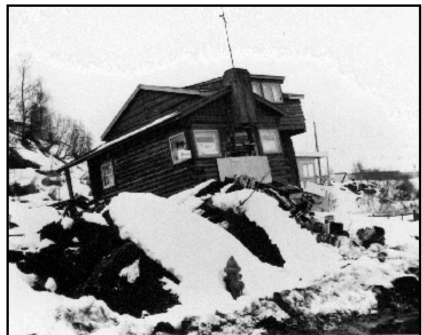
Pressure ridge at toe of L Street slide, Anchorage, 1964 Alaska Earthquake
