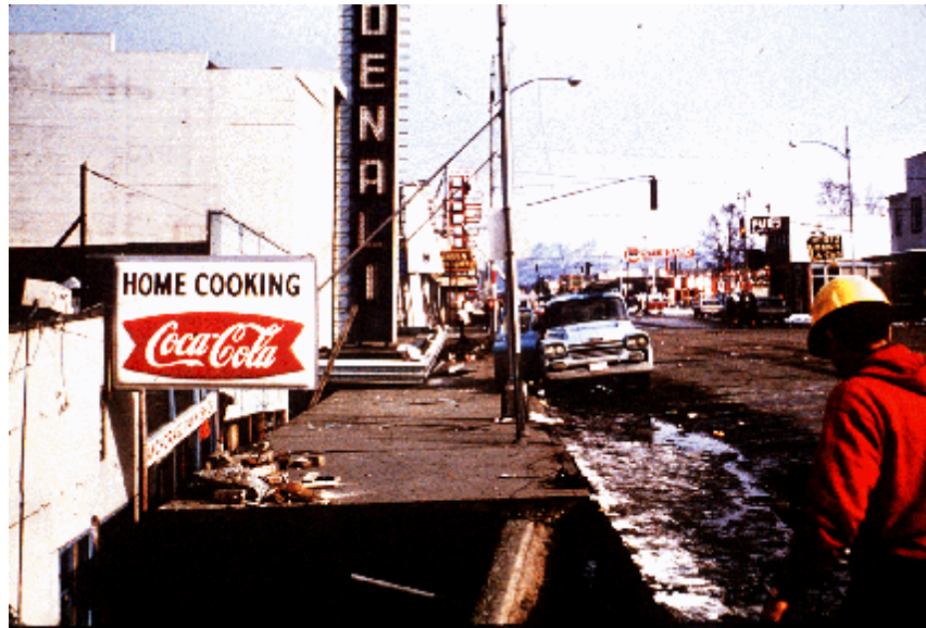
Photo 1.2 The marquee of the Denali Theater, which was in the graben of the Fourth Avenue landslide in Anchorage, subsided until it came to rest on the sidewalk in front of the theater, which was on ground that was not involved in the landslide. Source USGS.
