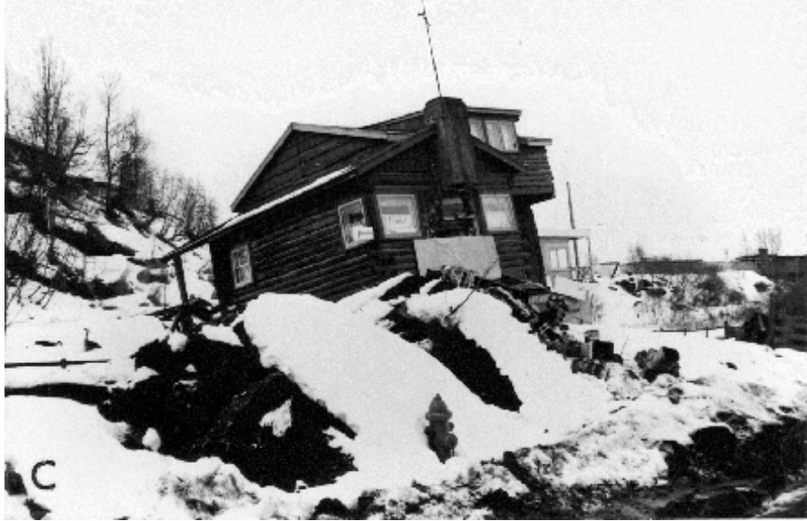
Photo 1.4 House displaced by compressional ridge formed at toe of L Street landslide. Source USGS.
