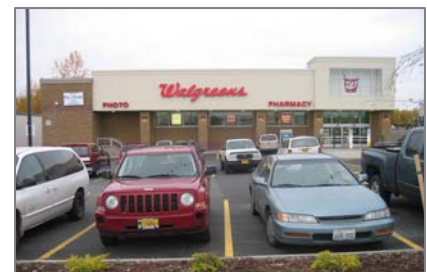
Walgreens at West Dimond Blvd.
