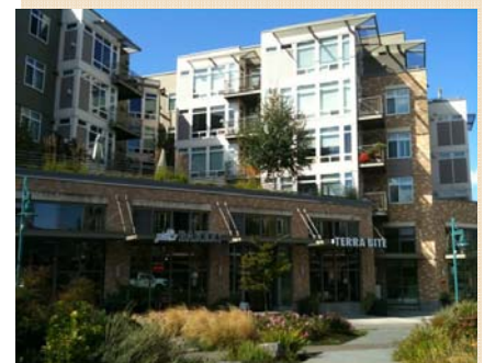
Commercial/Residential Mixed-use Example from Kirkland, WA
