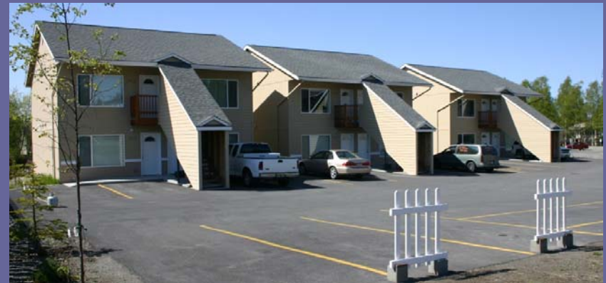
Lack of walkways or landscaping
