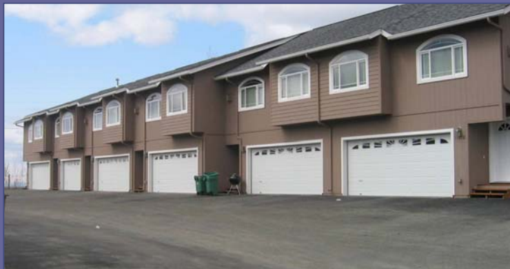
Absence of landscaping between driveways
