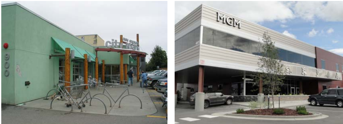
City Market's seating area and MGM Medical Office's entry plaza both comply
