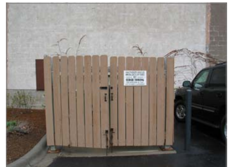
Above, sight obscuring gates are required for dumpsters in Minneapolis, MN.
