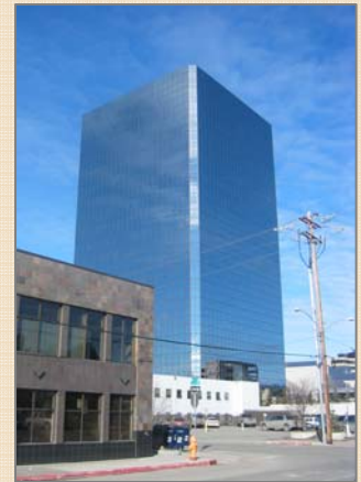
High rise designs do not respond to Anchorage’s local climate conditions can have severe wind and shadowing effects on the neighboring properties and public streets.
