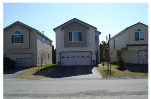
Estimated width of houses above: 24-feet. Garage door: 16-feet, or 67% of the façade. Provisionally adopted Title 21 allows 60%.
