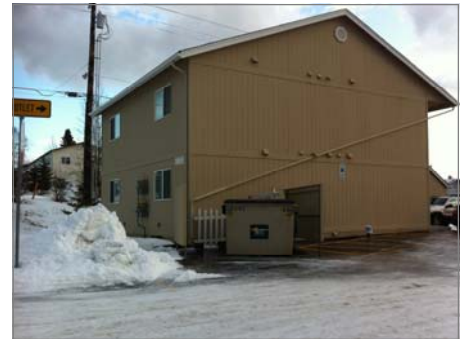
Without a screening enclosure and gate, this street-facing dumpster is what greets residents as they pass by this infill project in their longstanding neighborhood on W. 82nd Avenue at Jewel Lake Road.
