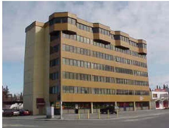
Woronzof Tower – 7 stories / 75 feet high
