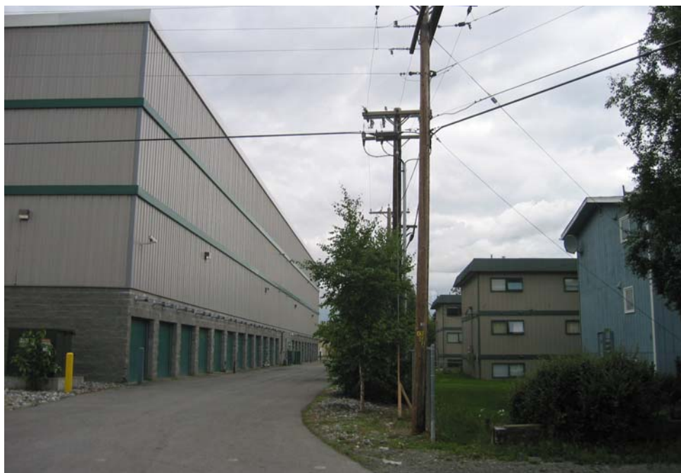
Tudor Storage building backs up close to the south property line of a residential area.
