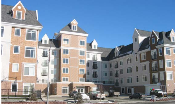
Park Plaza II has a floor-area-ratio of 1.6, 20% less than the maximum allowed bulk in R-4
