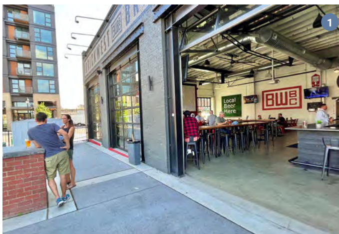
1. Downtown Spokane adaptive reuse project - exterior doors were added to connect the space to the outdoors. | 2. Example for a former auto shop converted to a restaurant. | 3. Example of a legacy storefront in Spokane's Hillyard District converted to a brewery/coffeeshop.
