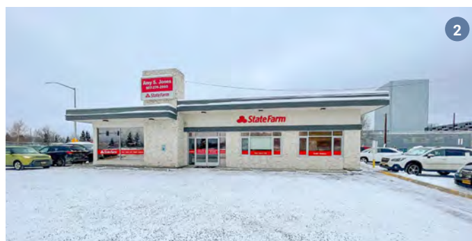
1. View of the existing parking lot next to the Alaska Oil and Gas Conservation building with the former Nordstrom store in the background. | 2. View of the existing office/commercial building at the corner of C Street and 9th Avenue. Future demolition, redevelopment, and adaptive reuse activities on properties like these may warrant environmental studies and/or regulated building materials surveys.
