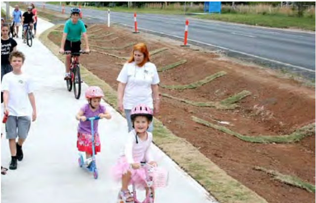
Swales at the edge of the pavement help to control and filter stormwater runoff, and can also function as snow storage areas in winter months. They can also act as a buffer between pedestrians and vehicular traffic.
