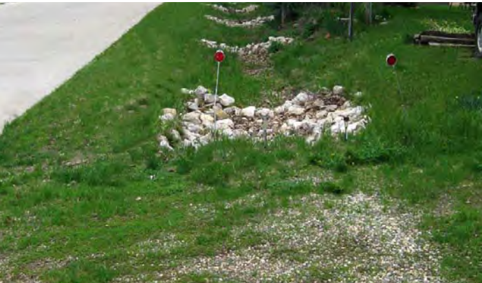
Swales at the edge of the pavement help to control and filter stormwater runoff, and can also function as snow storage areas in winter months. They can also act as a buffer between pedestrians and vehicular traffic.
