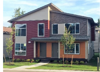
Good site access for pedestrians.
