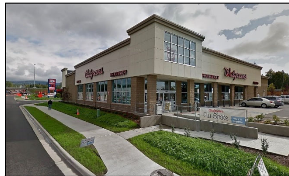
Commercial development with pedestrian-supportive street frontage.
