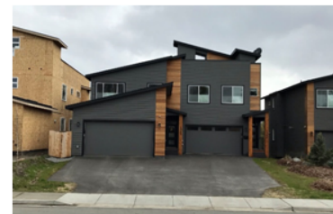
Example of sidewalk slope on new driveway curb cut.
