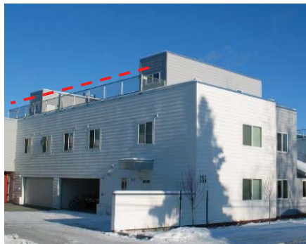
Transparent railing on left and solid parapet at right. Roof access enclosures in both.
