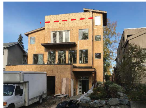
Transparent railing on left and solid parapet at right. Roof access enclosures in both.
