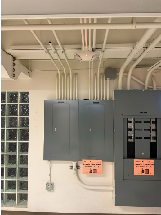
Figure 12 Existing MDP, existing Panels A and B
