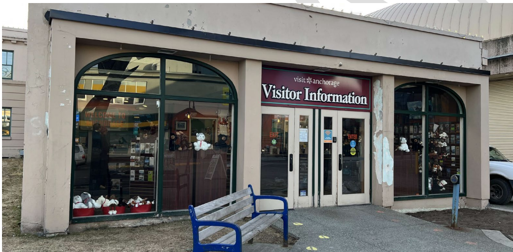
Figure 4 View of west end of building
