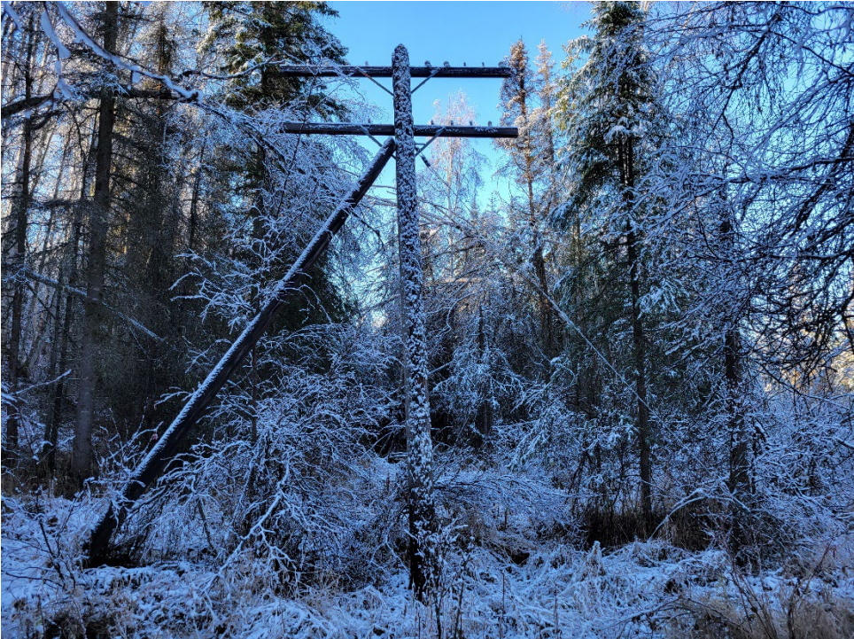
Figure 5. Pole with support beam and guy wire.
