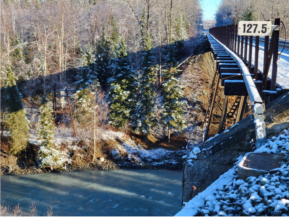
Figure 4. Pole near ANC-00099.
