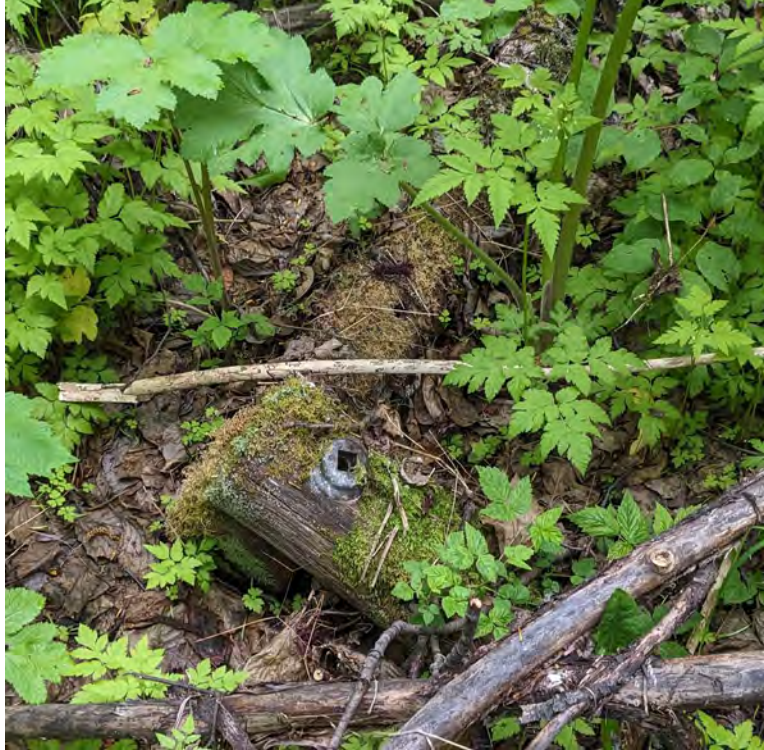
Figure 4. Fitness Structure #1; Connected beams
