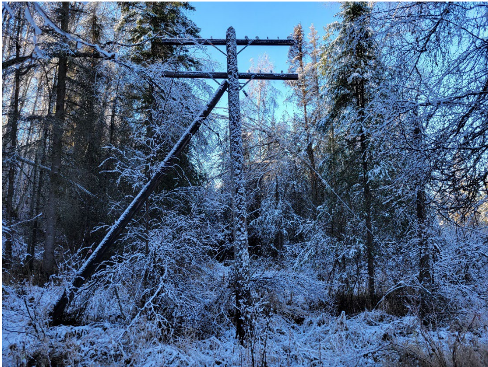
Figure 5. Pole with support beam and guy wire.
