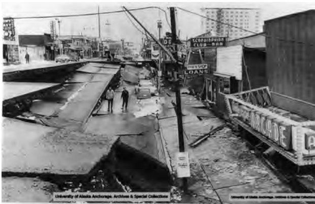
Figure 4. 4th Avenue after the 1964 Good Friday Earthquake, Anchorage, Alaska. Ruth A.M. Schmidt papers, University of Alaska Anchorage, uaa-hmc-0792-b4-f32-3.
