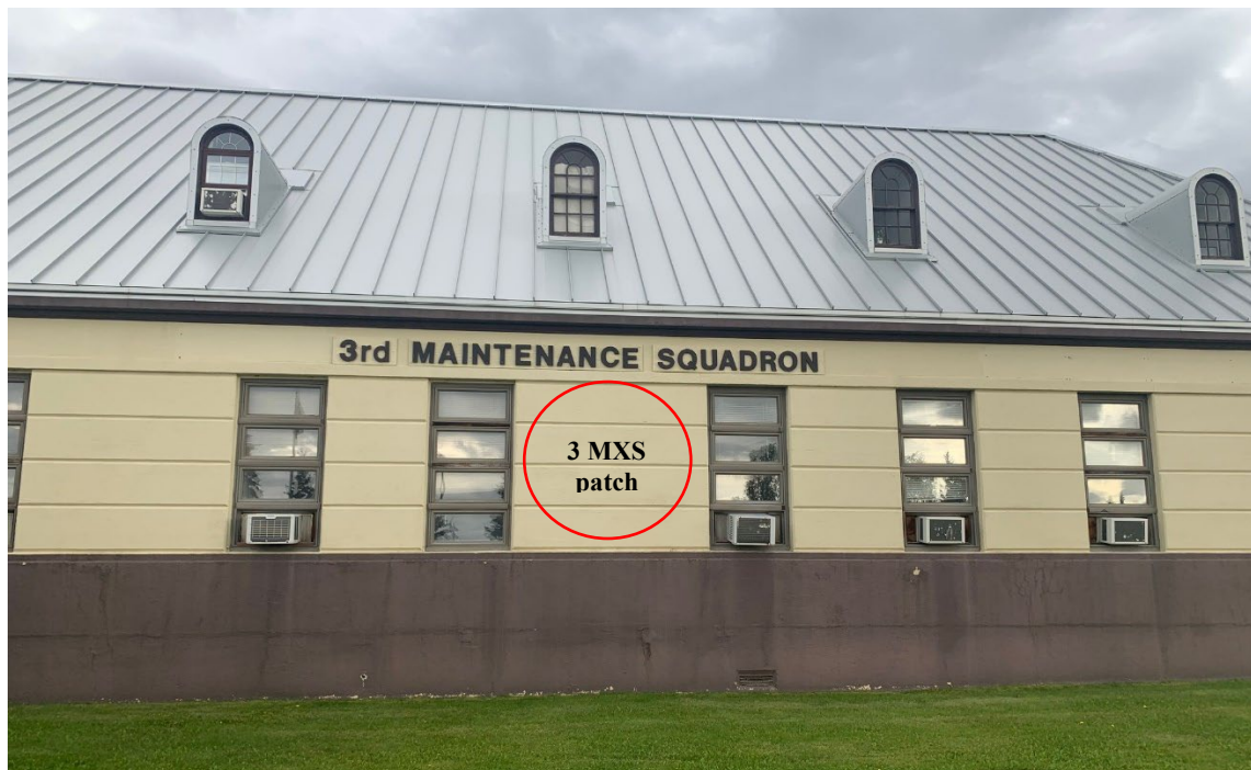
Figure 2. Building 11540 with placement of unit patch indicated.
