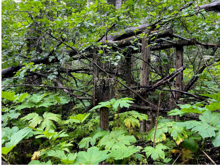
Figure 8. Fun N Fitness Trail™ Fitness Structure #2; Overhead Traverse (north facing)
