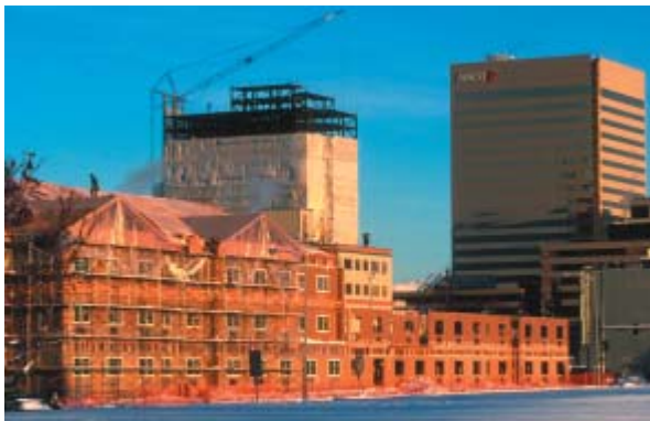
New hotel construction in downtown Anchorage
