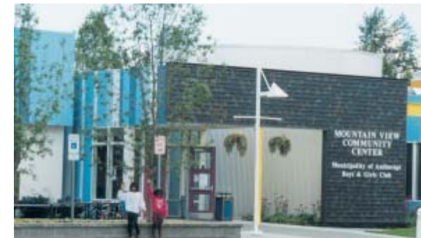
The newly renovated Mountain View Community Center is an example of a project made possible by neighbors helping neighbors.
