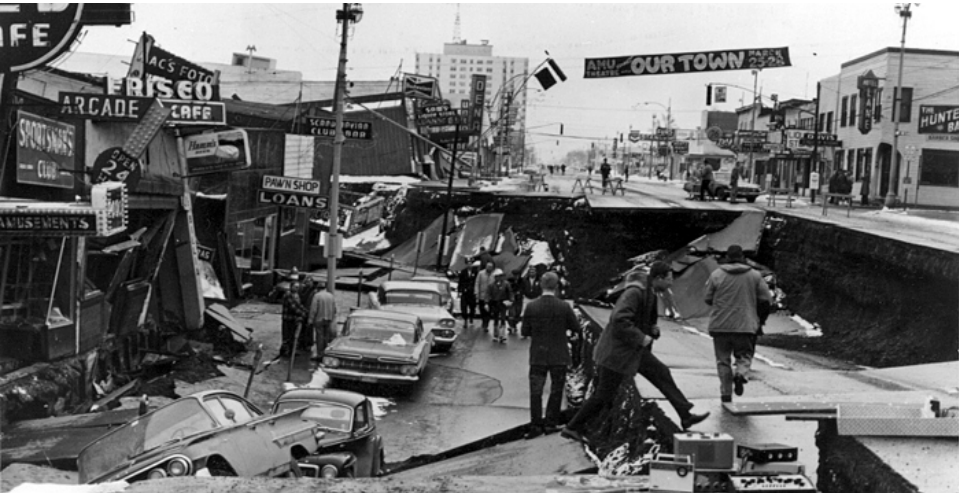
Seismic Ground Failure- 4th Avenue Slide
