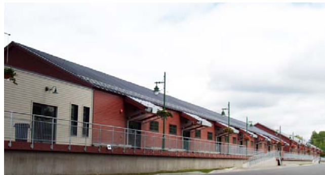
Newly renovated Alaska Railroad buildings
