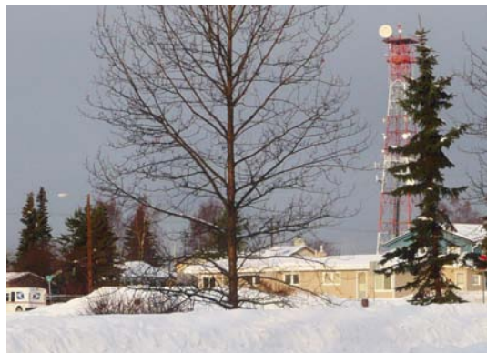
View of the wireless tower in Government Hill
