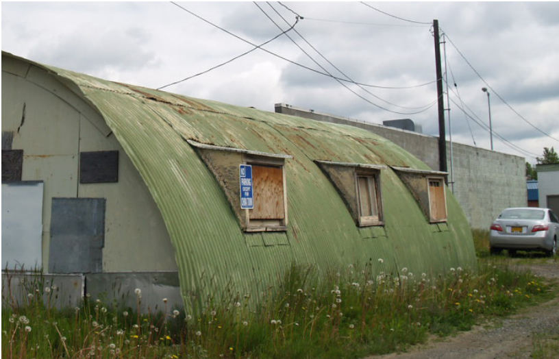
One of the original quonset hut structures
