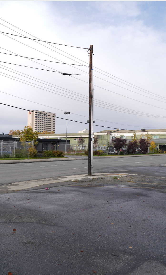
Utility Pole in Sidewalk.
