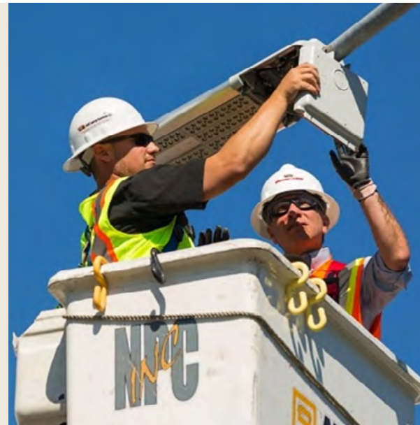
On Mar. 28, 2017, Mayor Ethan Berkowitz joined an M&O crew to install a new LED street light and "smart" controller node."
