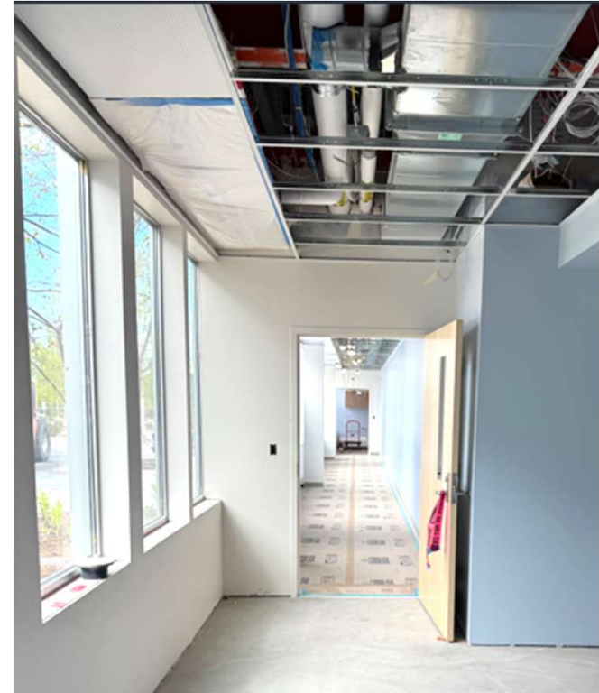
Passageway connecting services
