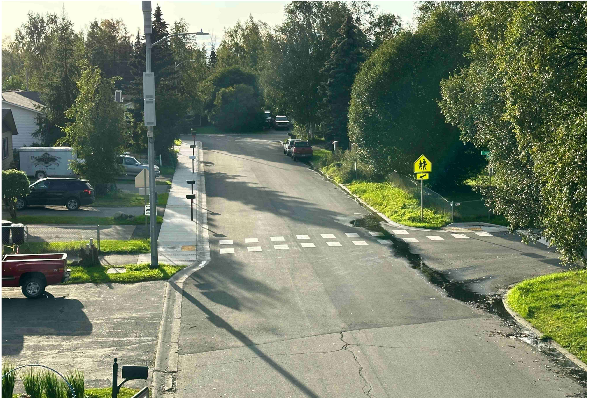
New Crossing at Lionheart Drive/Fireoved Drive and New Sidewalks on Lionheart Drive (Wonder Park Elementary School)
