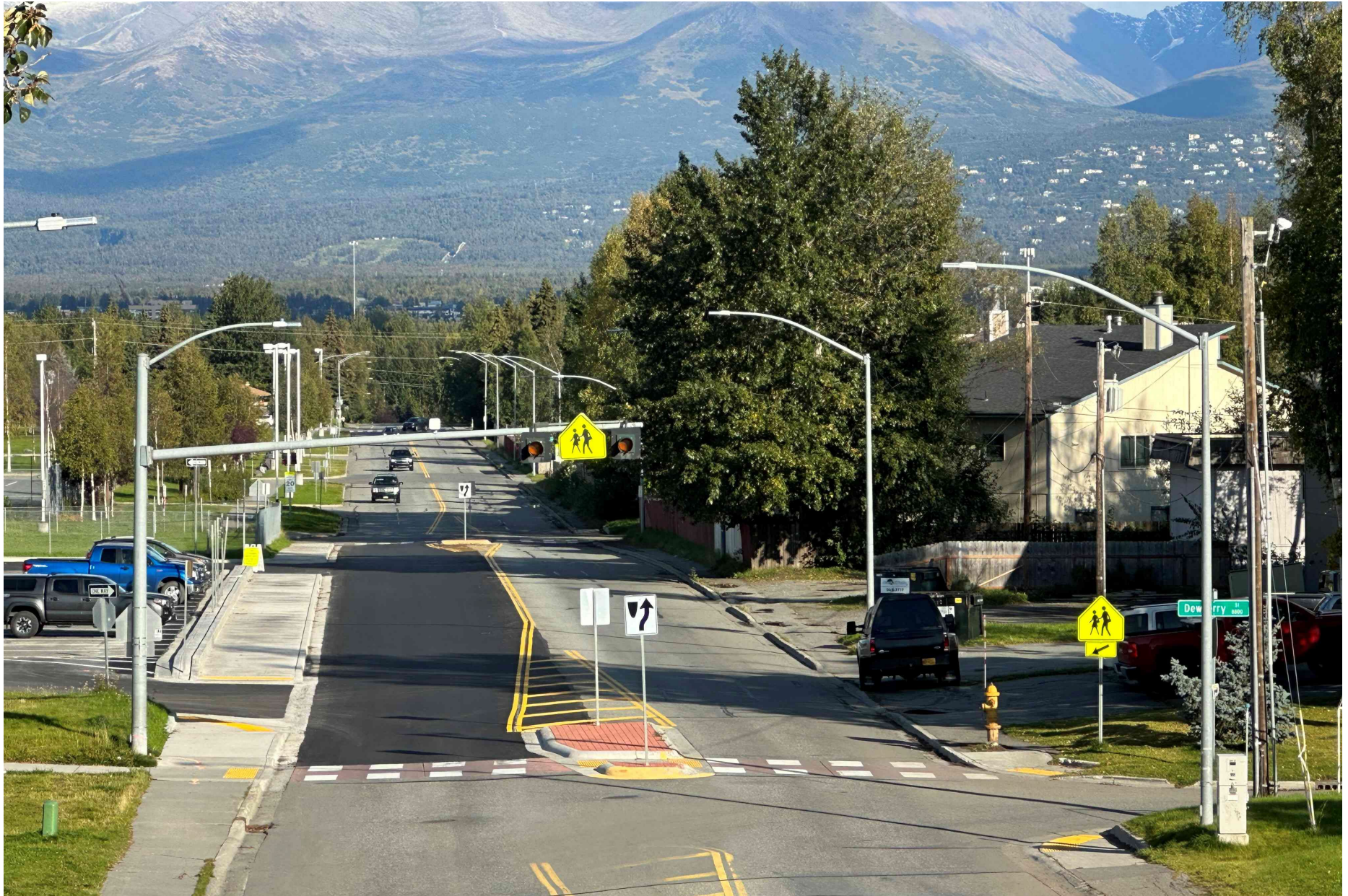
Replace Sidewalk on 88 th Avenue (Chinook Elementary School)
