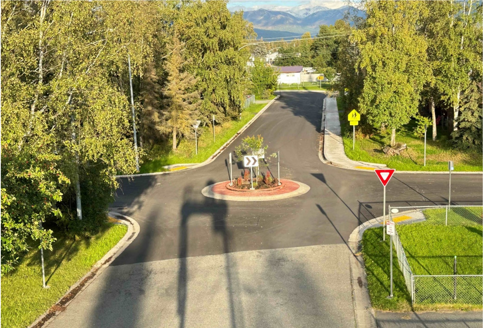
Mini Traffic Circle at Kenai Avenue/Stewart Street and New Sidewalk on Kenai Avenue (Wonder Park Elementary School)
