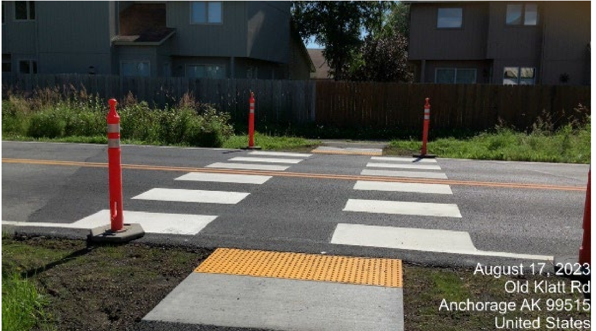
Intersection Curb Ramp and Sidewalk Repairs at Old Klatt Road (Klatt Elementary School)
