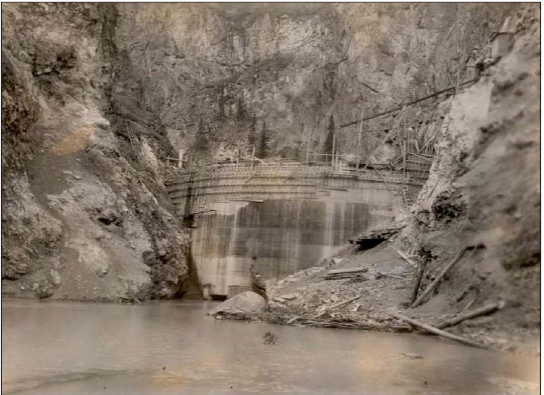
Figure 12. Upstream face of diversion dam under construction.
