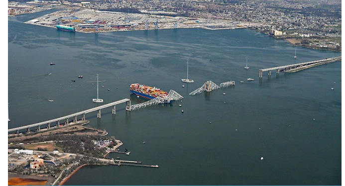
Francis Scott Key Bridge Port of Baltimore 3/24
