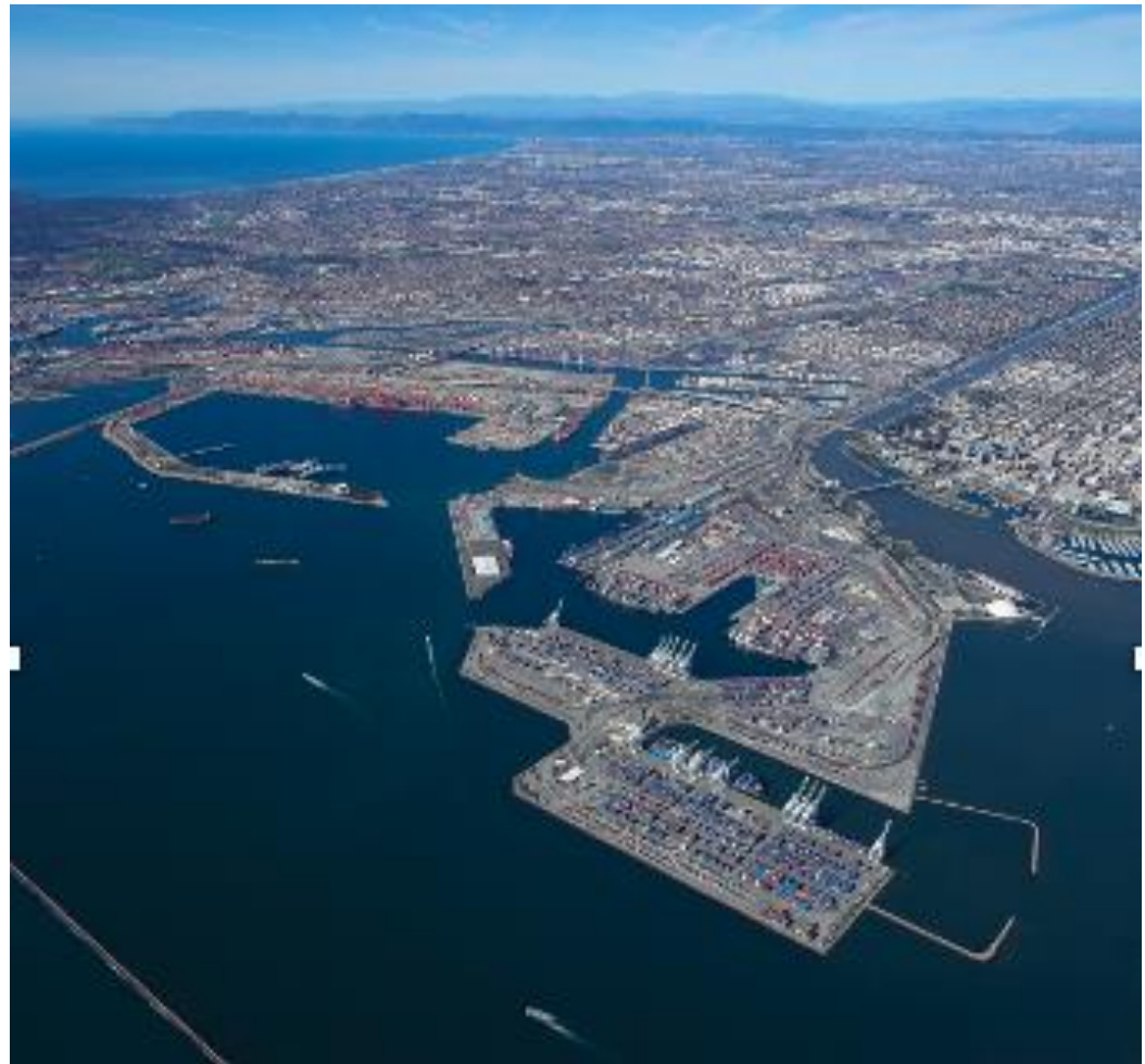
Aerial view of Port of Long Beach
