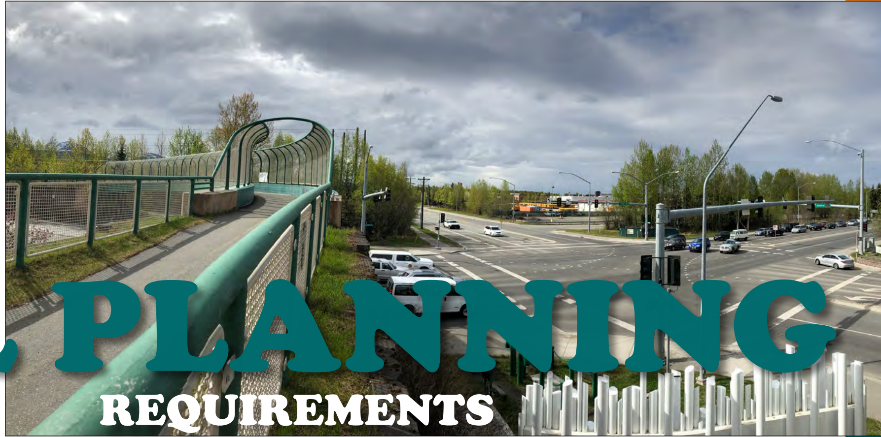
Intersection of Tudor Road and Elmore Road with multiuse trail overpass – courtesy of AMATS/Municipality of Anchorage.
