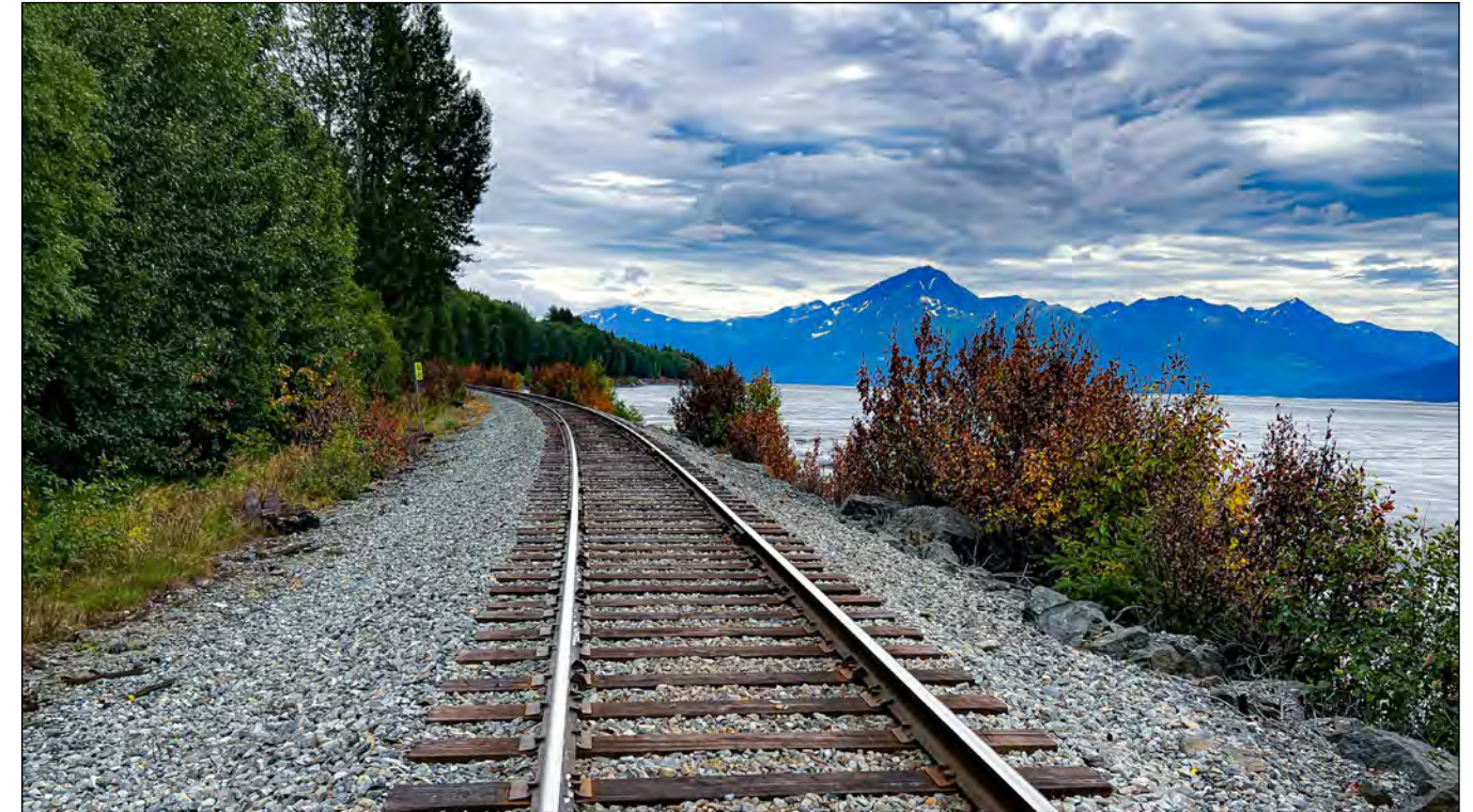
Alaska Railroad along Turnagain Arm.
