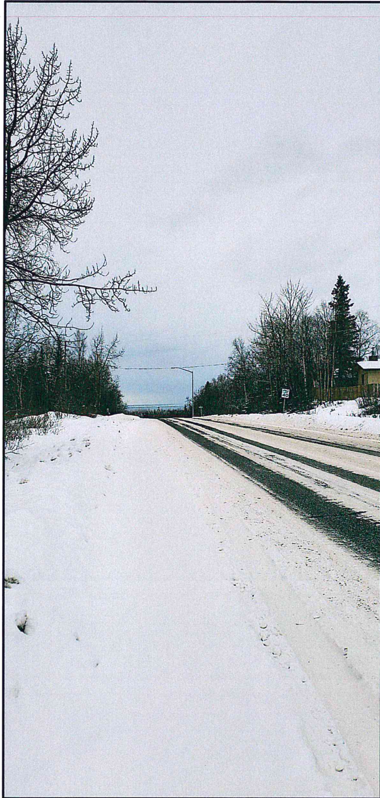
Proposed Intersection Looking West (Measured Sight Distance = 375 Feet)
