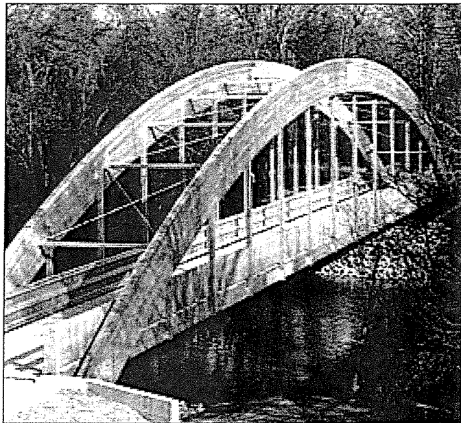
The Tar River trail bridge in Rocky Mount, North Carolina features glued laminated arches.
