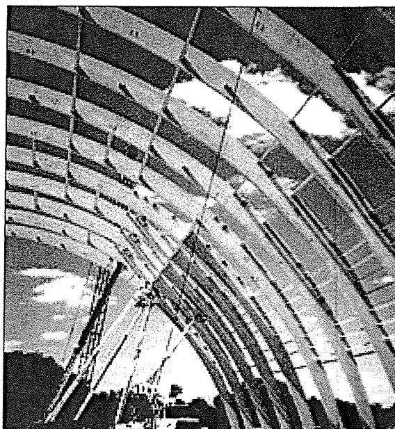
Glulam arches support the roof of the Chicago Bears practice facility in Lake Forest, Illinois.
