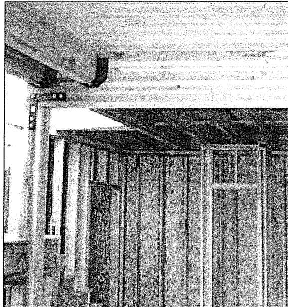
Glulam columns and headers provide primary support in this condominium construction.
