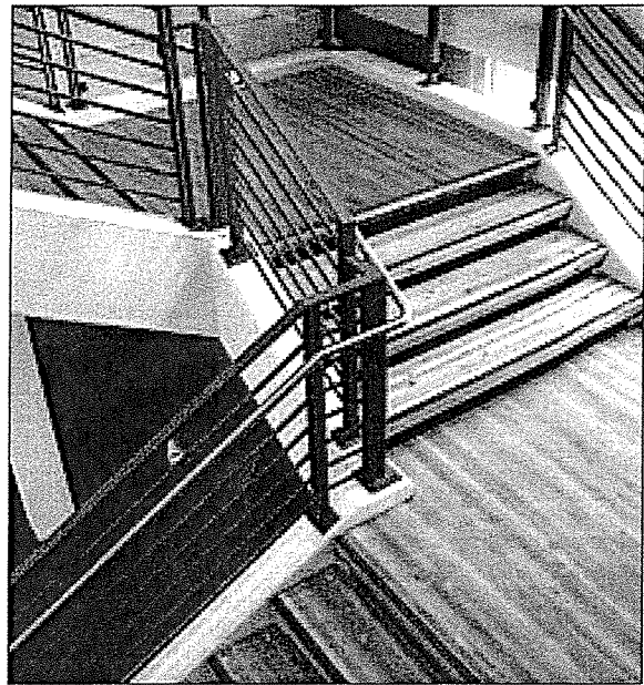
Durable glulam forms a resilient stair tread.
