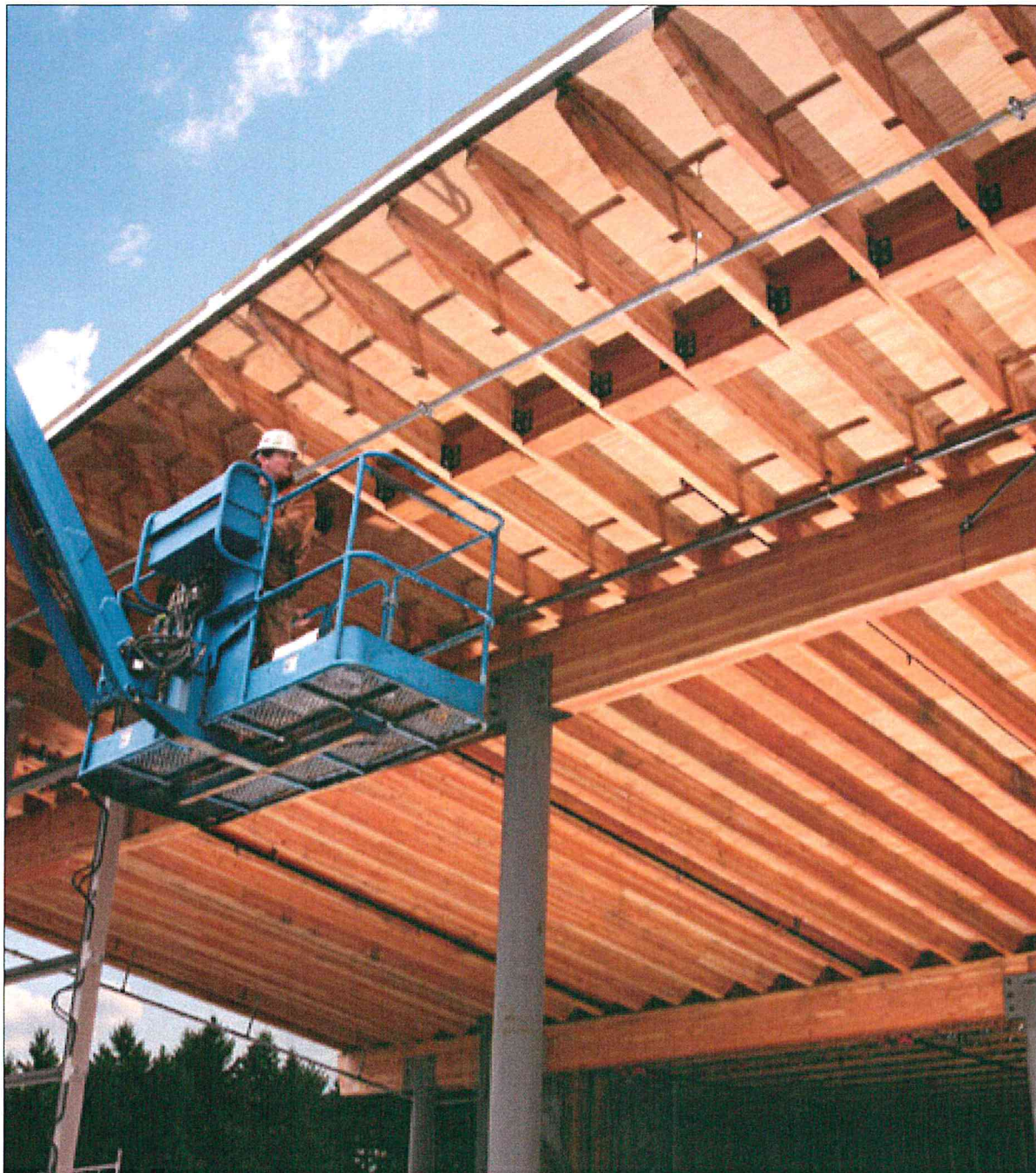
Architectural-grade glulam supports the atrium in the Garfield Commons building at Pacific Lutheran University in Tacoma, Wash.
