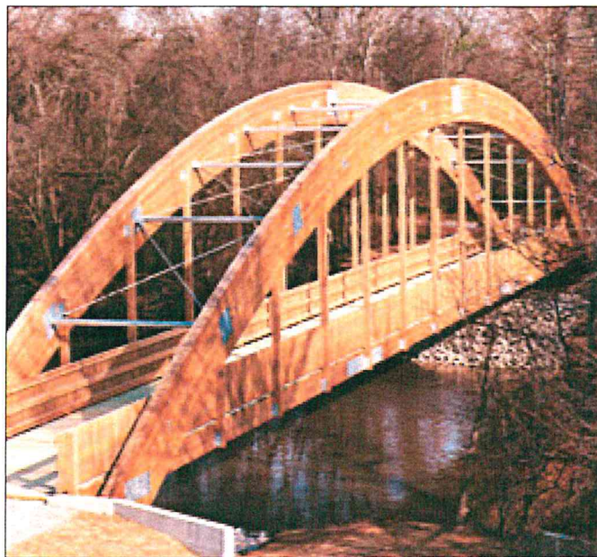
The Tar River trail bridge in Rocky Mount, North Carolina features glued laminated arches.
