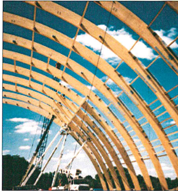
Glulam arches support the roof of the Chicago Bears practice facility in Lake Forest, Illinois.
