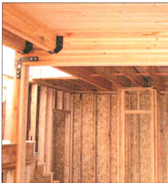
Glulam columns and headers provide primary support in this condominium construction.
