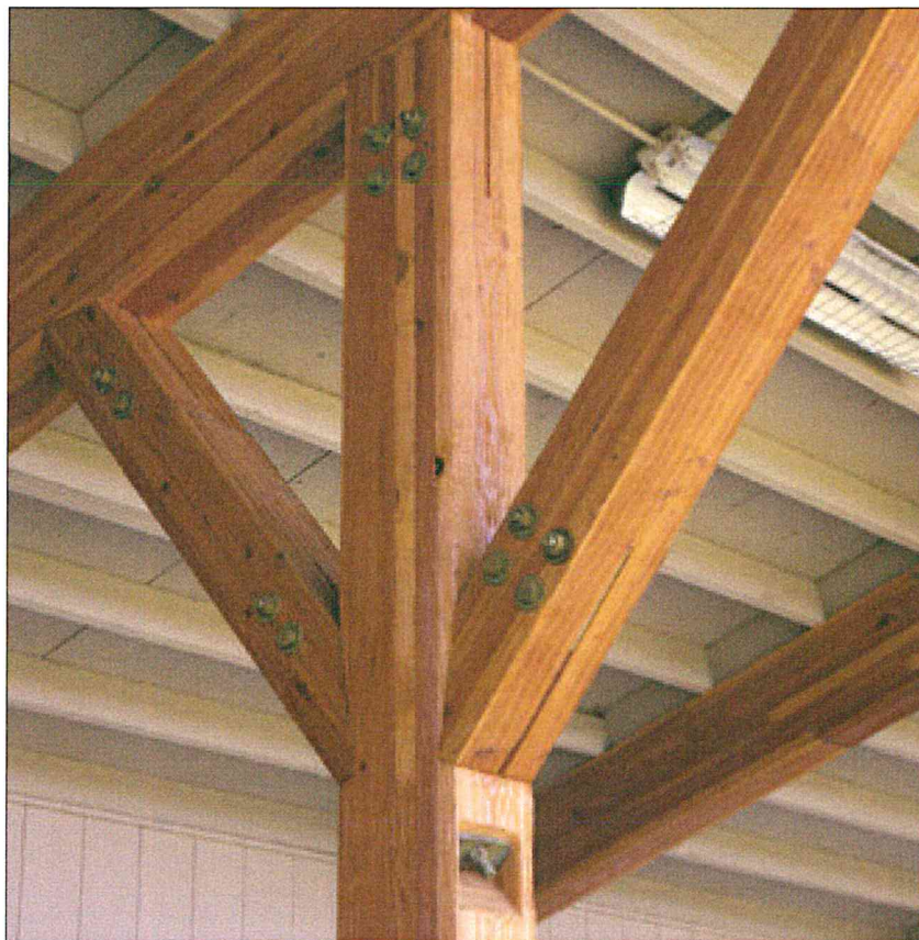
These glulam members use notches and hidden connectors, resulting in a clean, uncluttered design.
