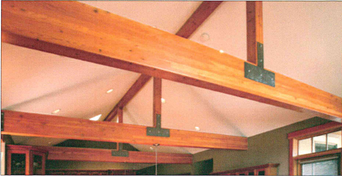
Exposed glulam beams in the ridge and intermediate supports for this condominium residence provide both visual drama and structural integrity.
