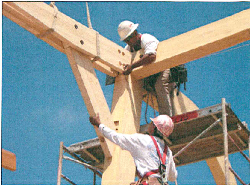
Holes and notches must be precisely located and detailed for architectural appearance and accounted for in the design of beam connections and column capacity.
