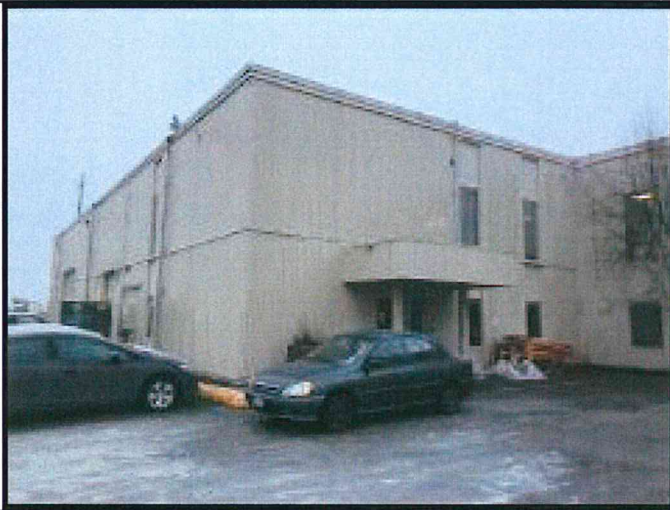
View northwesterly of main entrance into warehouse portion of the building.
