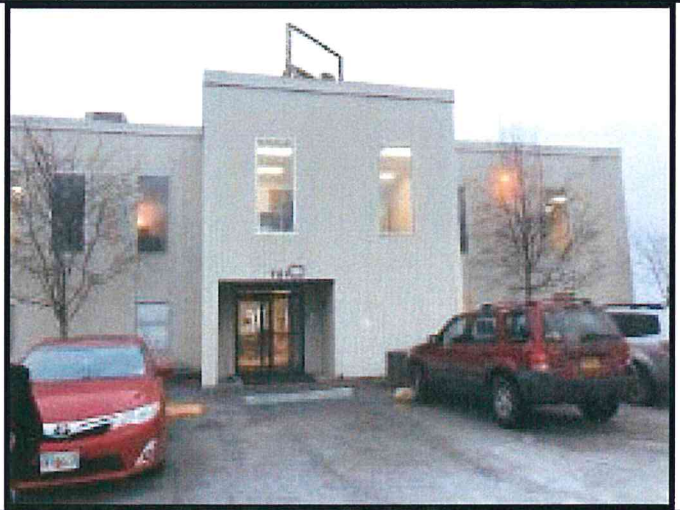
Looking north at the main entrance the office portion of the building.
