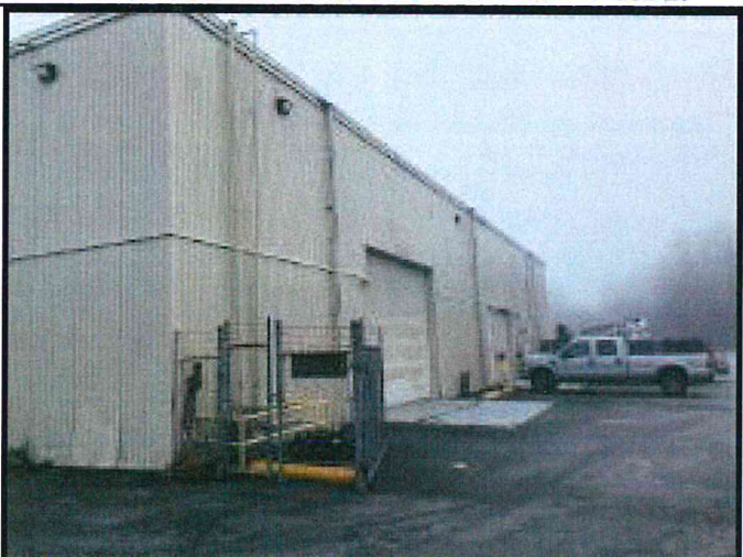
View northeasterly of front of the warehouse portion of the building.
