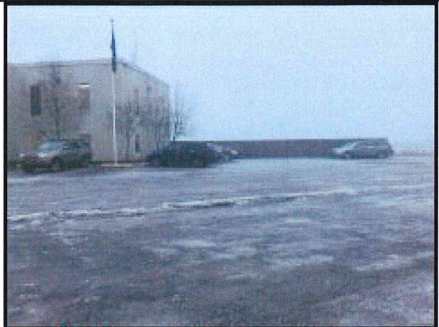
Looking north from/near the SEC.
