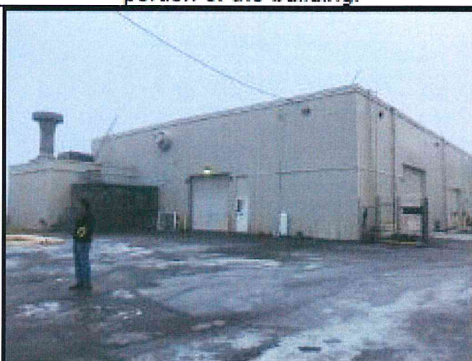
View northeasterly of the warehouse portion of the building.
