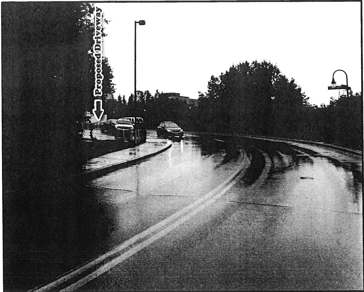
Figure 4 - Sight Distance to Driveway #1 through Parking Lot
