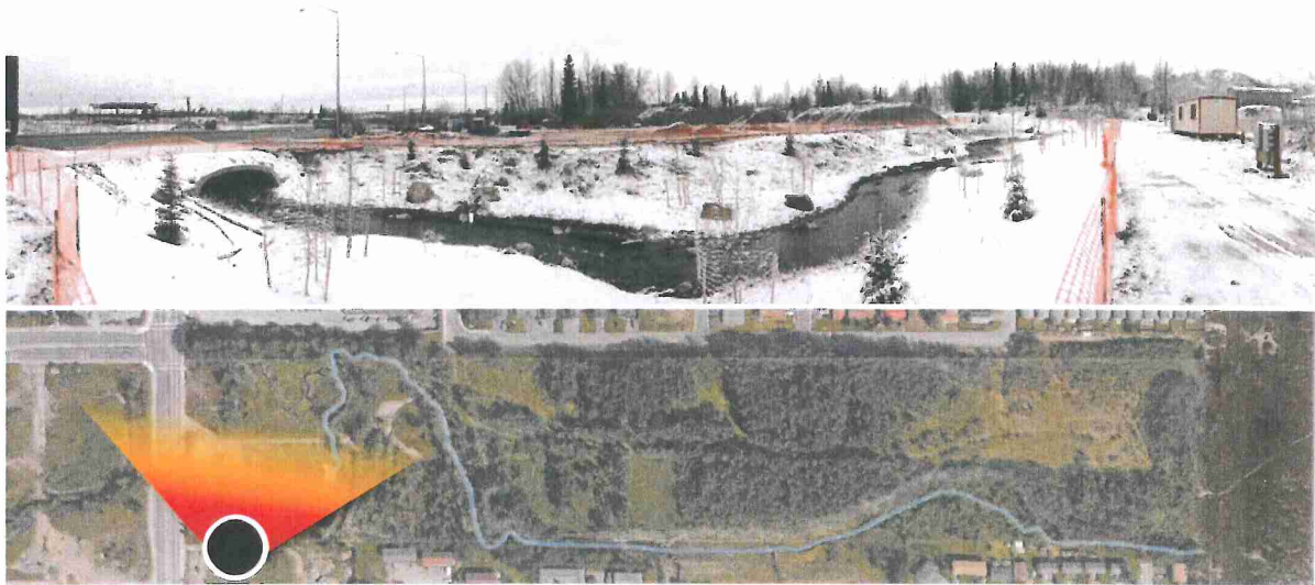
Existing conditions of Tract A and Chester Creek Realignment, facing north
