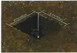
FIGURE 7-3. Hole prepared for tower base
