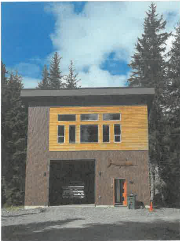
South Elevation (view from driveway)
