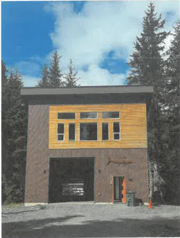
South Elevation (view from driveway)
