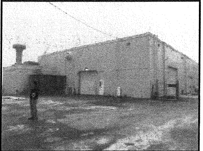
View northeasterly of the warehouse portion of the building.
