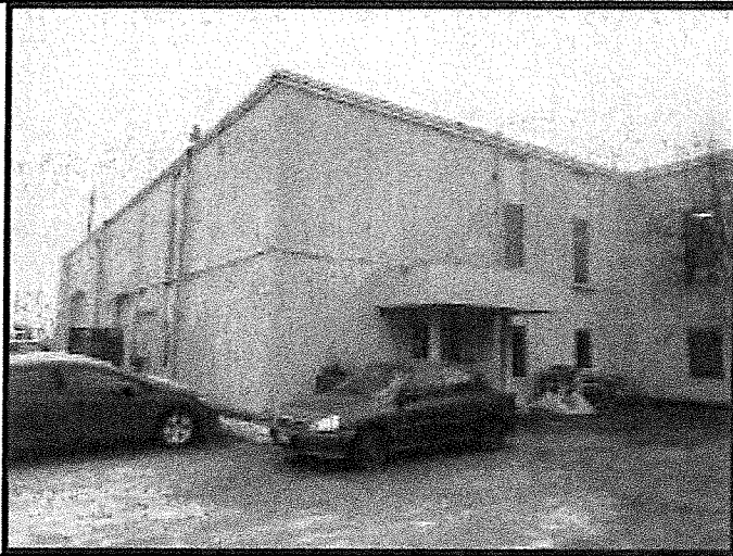
View northwesterly of main entrance into warehouse portion of the building.
