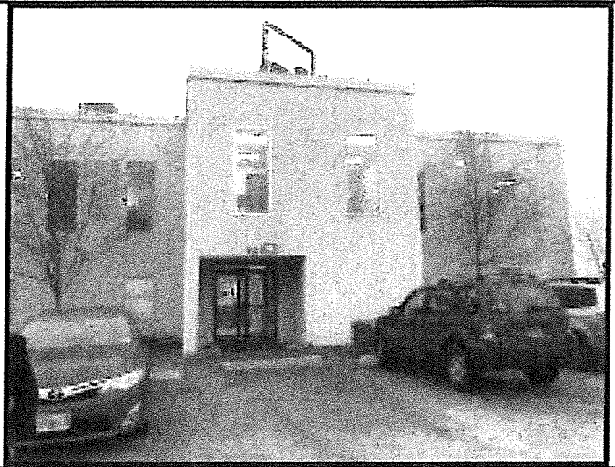
Looking north at the main entrance the office portion of the building.
