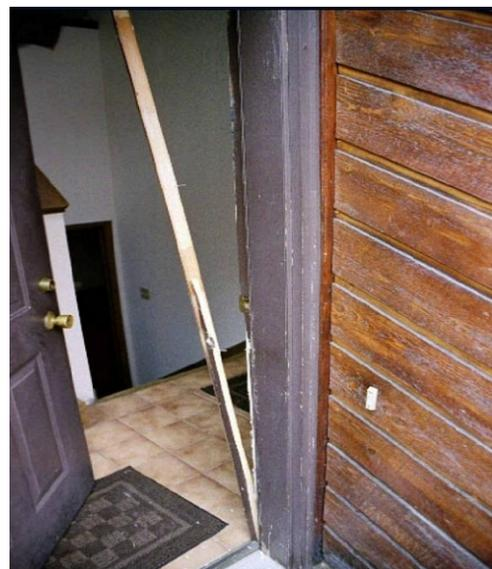
When someone kicks in a door, it's not the lock or the door itself that gives, it's the door jam. Replace all the screws in the strikeplates on the door jam with 3" screws, securing the door jam into the frame.
