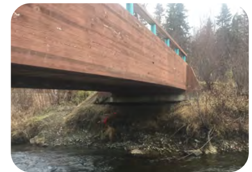
Existing Bridge (Exposed Foundation Looking North)
