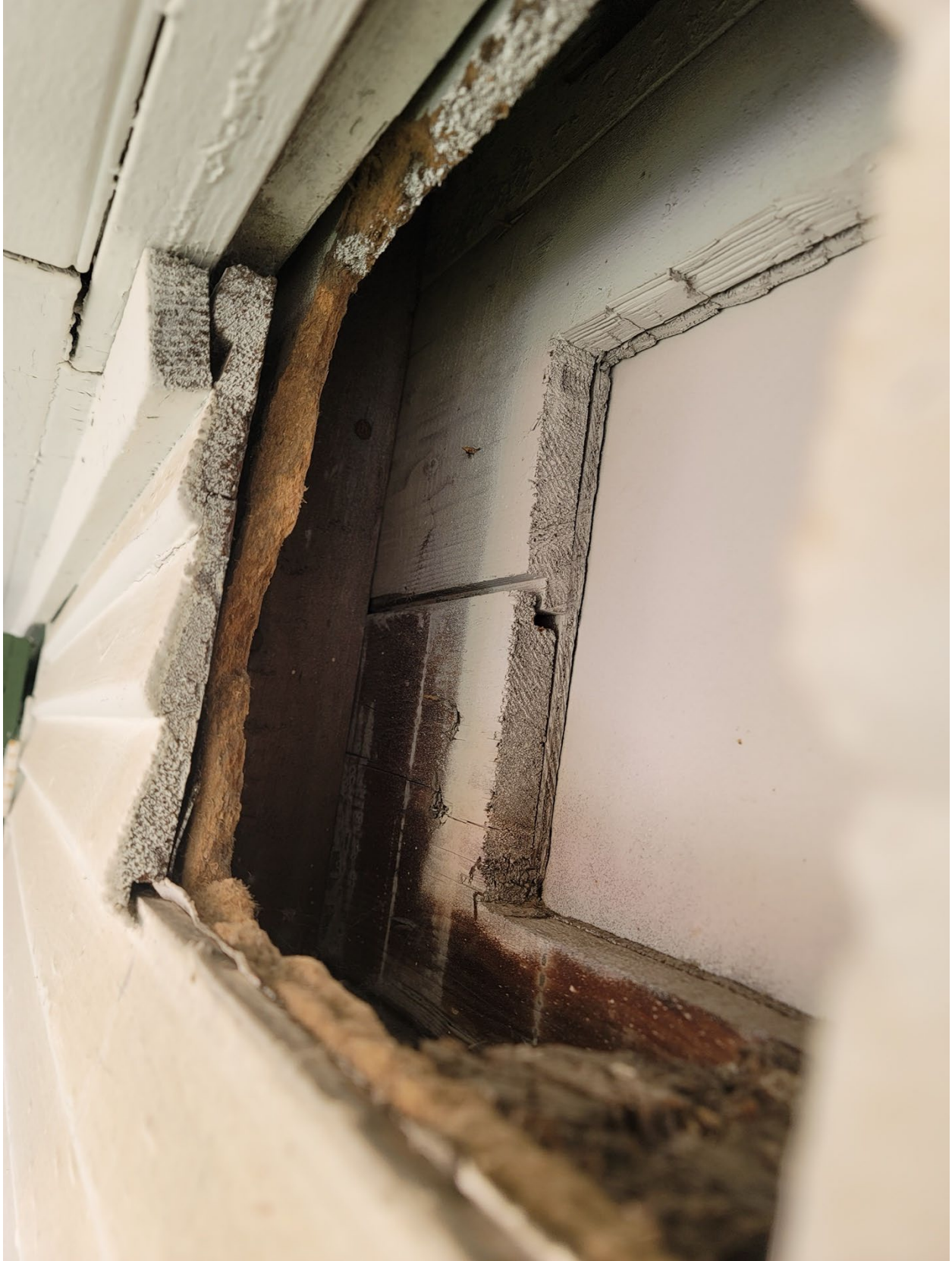
Figure 17. Detail photograph showing the current siding overlaying older siding layers on Building A (©TNSDS 2023).
