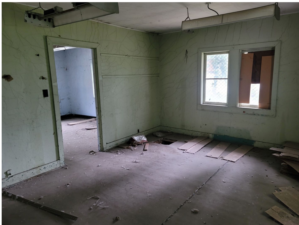
Figure 51. Interior of the northernmost rooms in Building A. The photograph shows the holes and cracks in the flooring and wall finishes (©TNSDS 2023).
