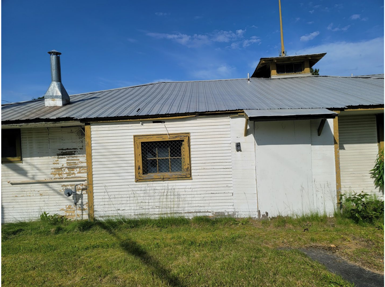
Figure 32. Detail photograph of the stairwell addition on the east façade of Building A. The awning over plywood covers the entrance that leads to the stop of the stairs from the exterior (©TNSDS 2023).
