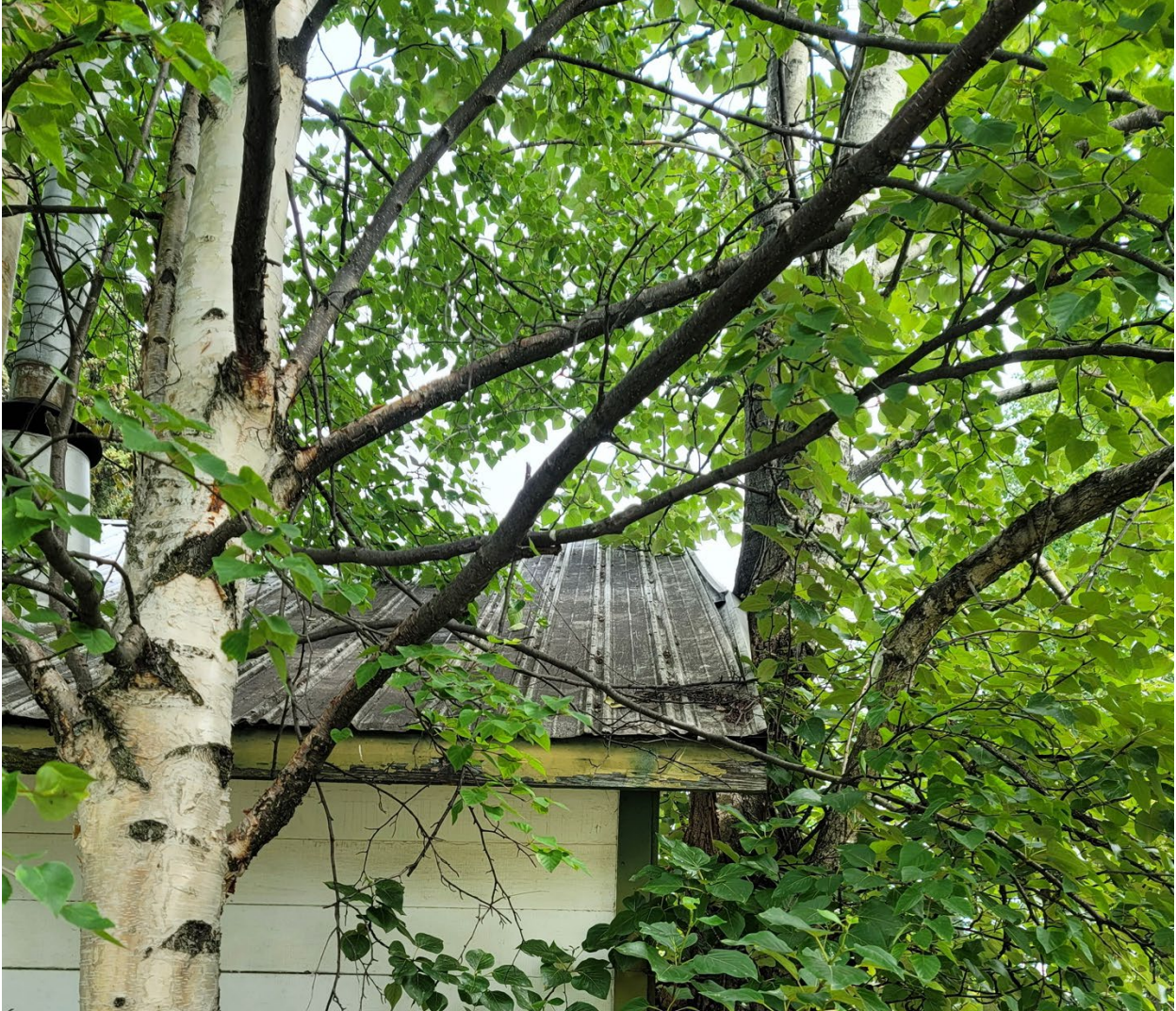
Figure 20. Detail photograph of Building C. The photo shows how the birch tree that has grown against the southeast façade of the building has begun to displace the roofing materials (©TNSDS 2023).
