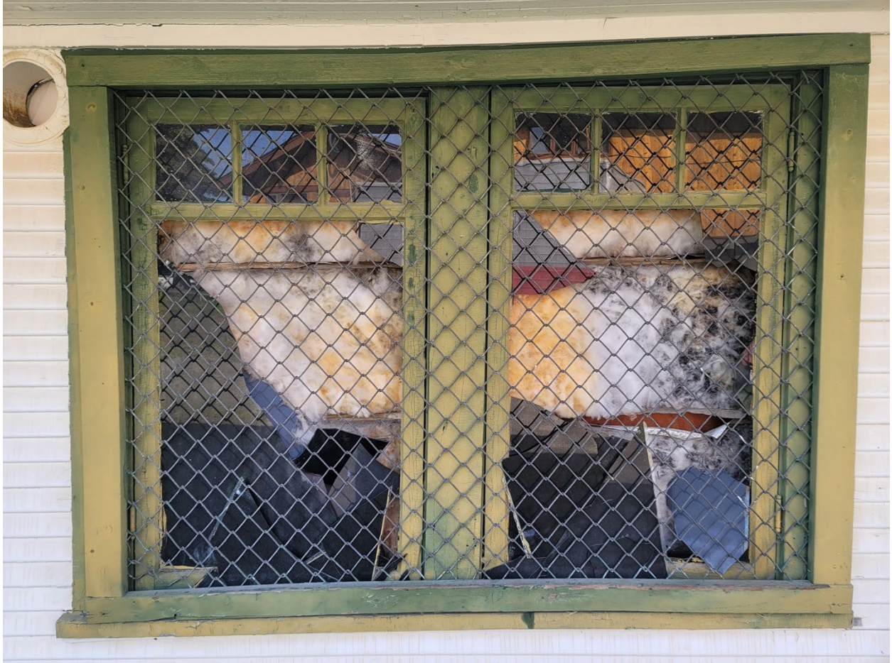
Figure 27. The southernmost window on the west façade of Building A. The photograph shows the broken glazing as well as the misalignment of the window framing due to the building's uneven settlement over time (©TNSDS 2023).
