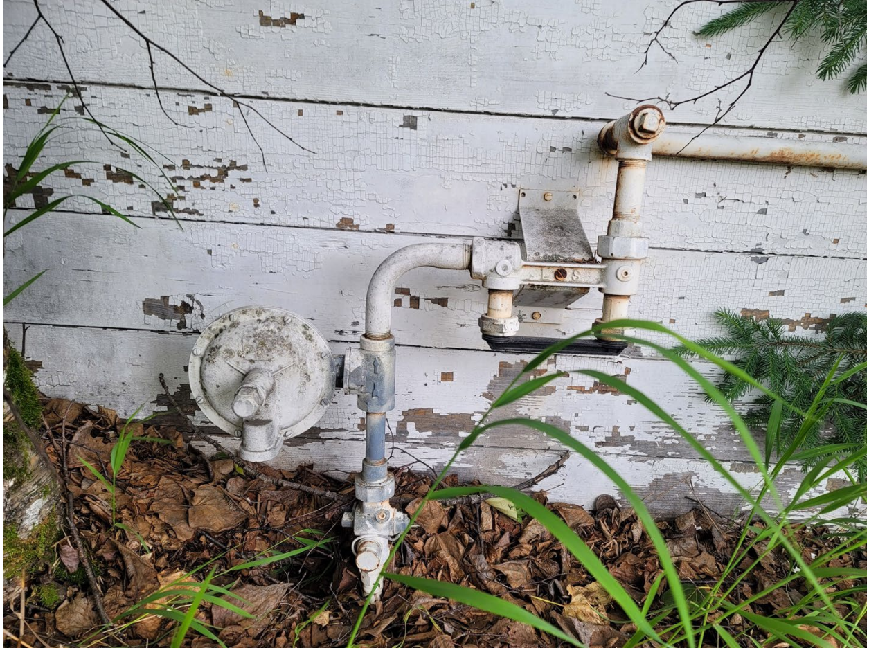
Figure 22. Detail photograph of the utilities installed on the southwest façade of Building C. The photograph shows the deterioration of the paint along the bottom boards of the building. It also demonstrates the crazing and cracking of the older paint as well as sections where the older paint has been removed and reapplied such that no cracking or crazing is present (©TNSDS 2023).
