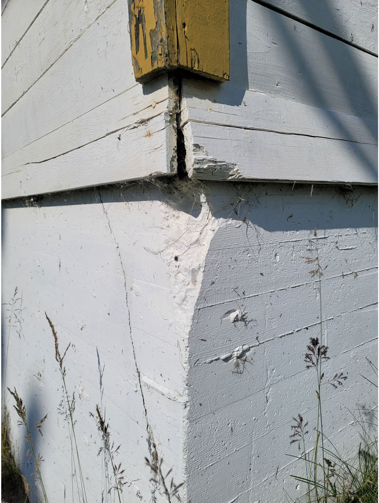
Figure 16. Detail photograph of the southeast corner of Building B. The photograph shows the concrete foundation, lap siding, and skirtboard and demonstrates the spalling happening to the foundation (©TNSDS 2023).
