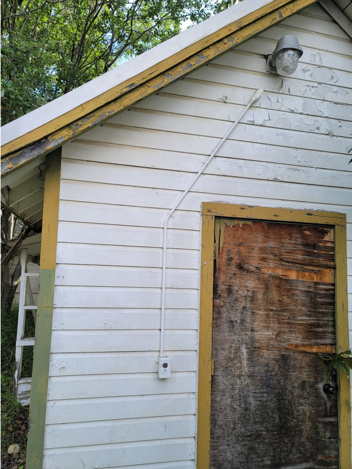
Figure 19. The southwest façade of the addition to Building B, showing the cracking, crazing, and peeling of the paint on the siding (©TNSDS 2023).
