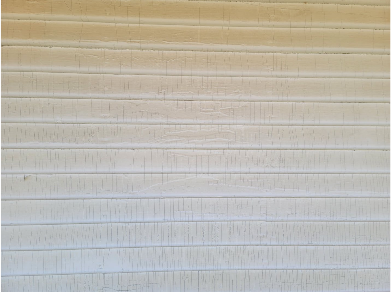
Figure 18. The wrinkling, crazing, and peeling in the paint on the west façade of Building A (©TNSDS 2023).
