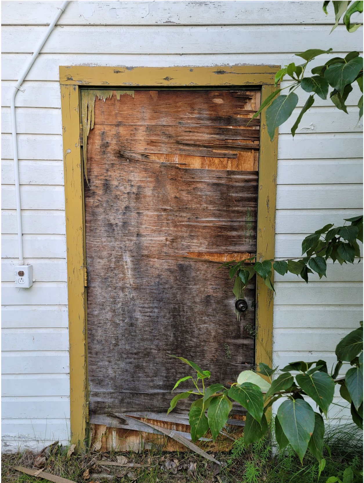
Figure 36. Detail photograph of the door in the southwest facade of the addition of Building B. The photograph shows the significant deterioration of the door material (©TNSDS 2023).
