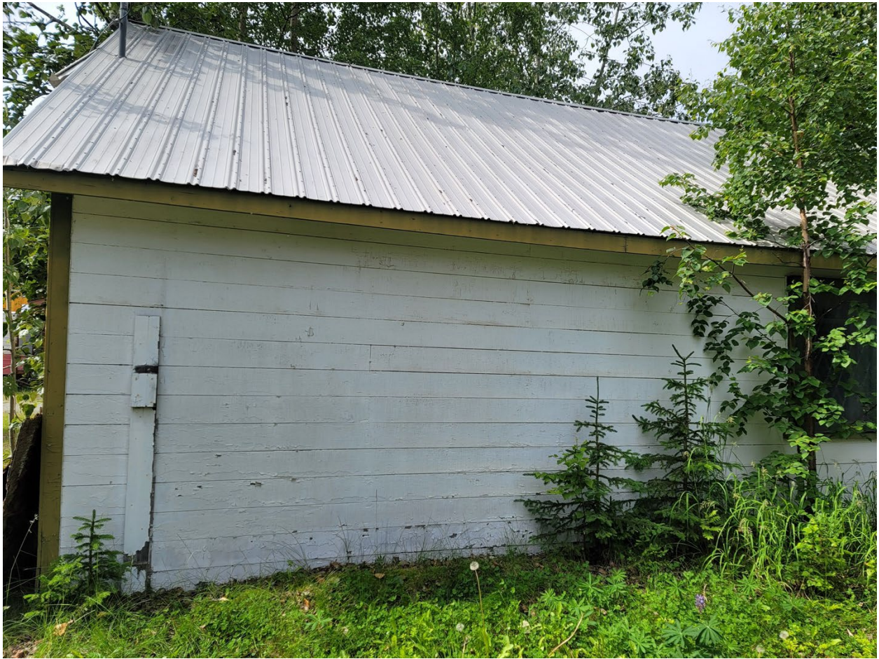
Figure 50. Photograph of the northeast façade of Building C, showing the onion corrugated polycarbonate or PVC roofing material (©TNSDS 2023).
