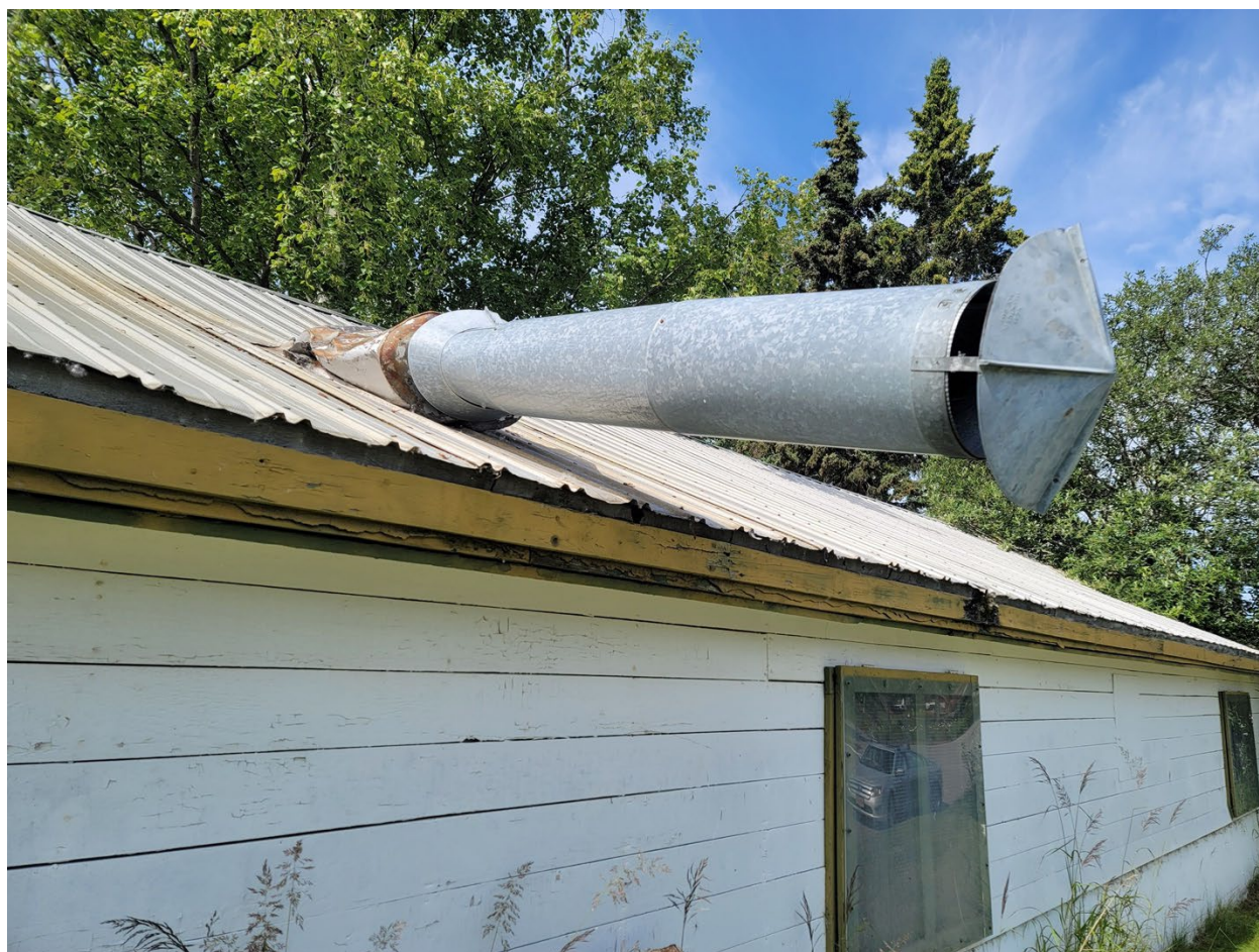
Figure 47. Detail photograph of the collapsed chimney on Building B (©TNSDS 2023).
