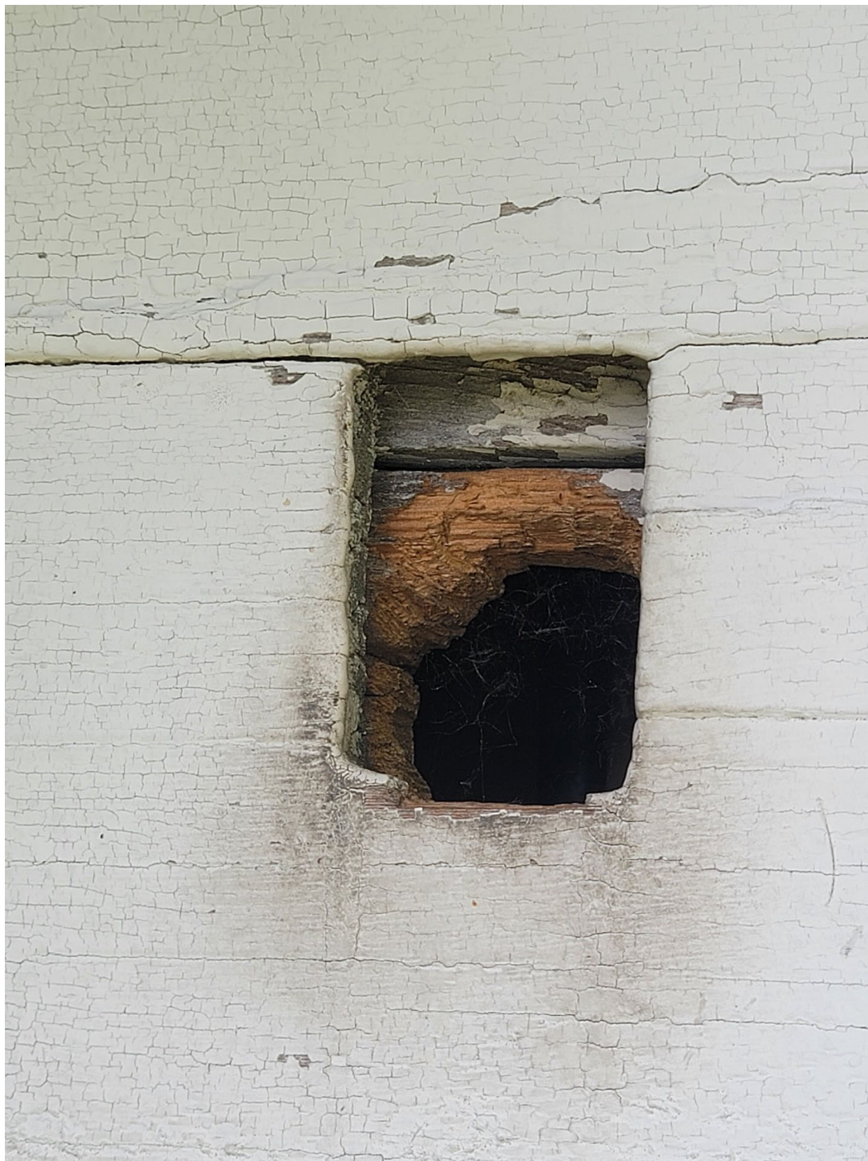
Figure 21. Detail photograph of an opening the siding of Building C, exposing the interior wood planks (©TNSDS 2023).
