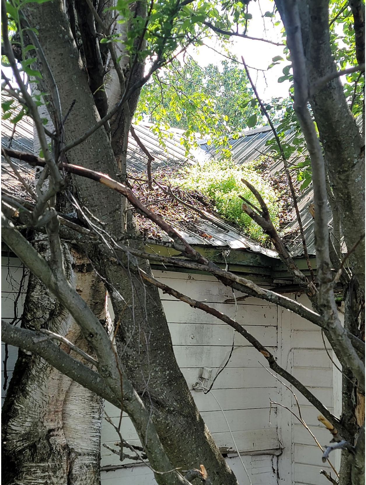
Figure 49. Detail photograph of the junction of the two sections of Building B. The photograph shows the roofing material, surrounding vegetation, and the vegetative debris growing on the roof valley (©TNSDS 2023).
