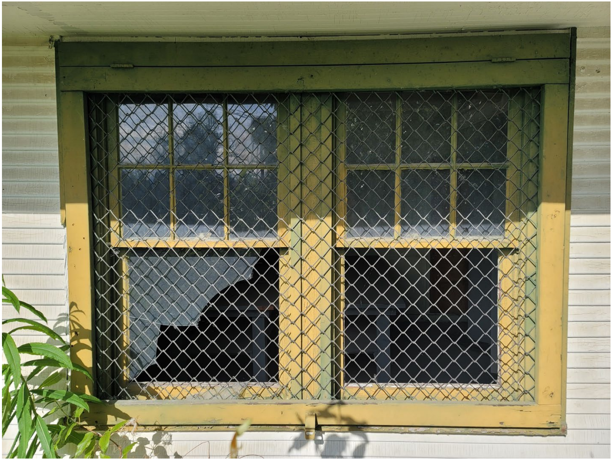
Figure 25. Detail photograph of the six-over-one sash windows in the east façade of Building A (©TNSDS 2023).
