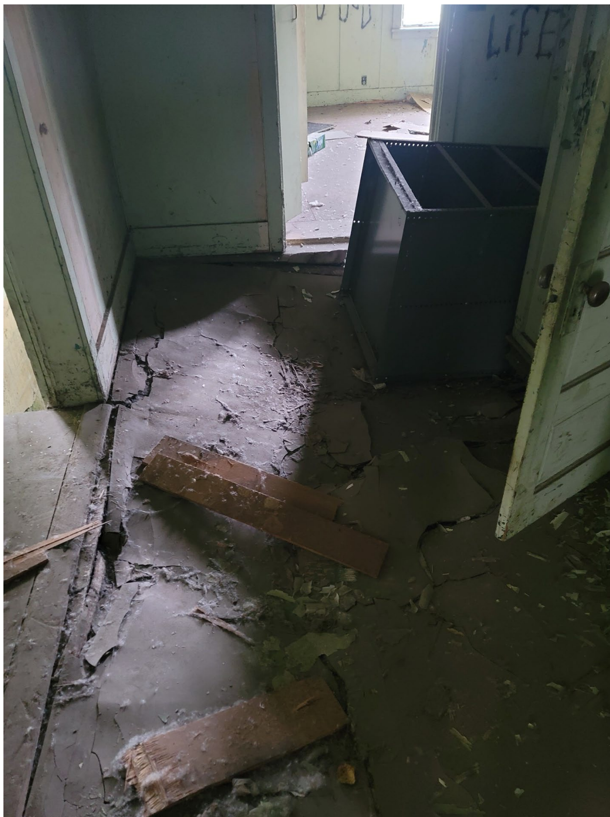
Figure 54. Photograph of one of the collapsed floors in Building A (©TNSDS 2023).
