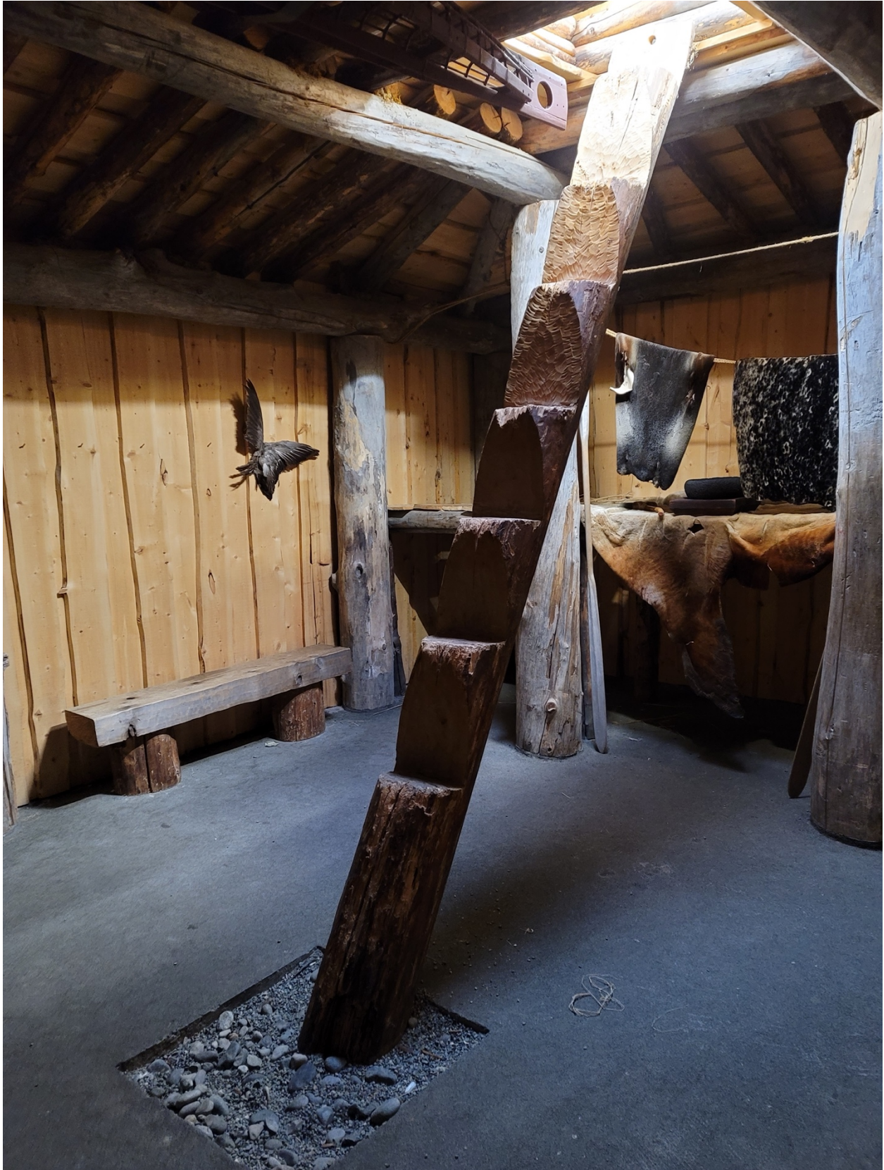
Figure 30. The interior of the western ulax, showing the timber ladder that would have provided traditional access to the ulax (©TNSDS 2023).
