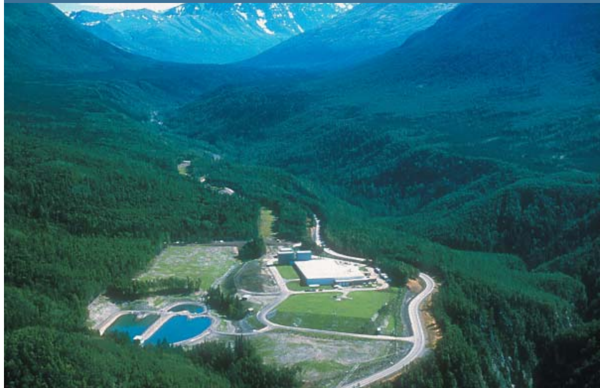
The Eklutna Water Treatment Facility supplies water to the Anchorage Bowl area.
