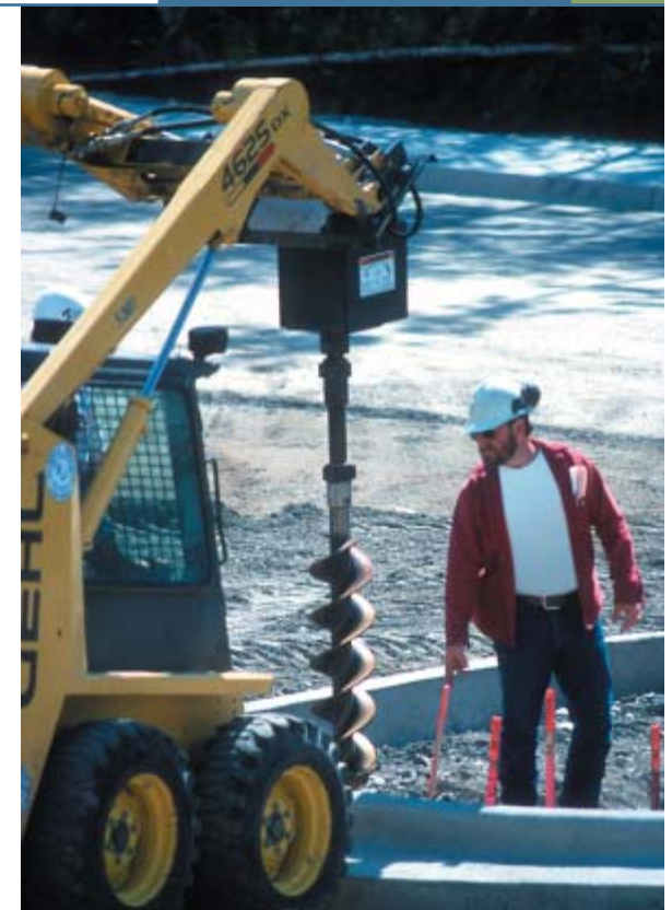
Construction accounts for 5.4 percent of Anchorage employment.
