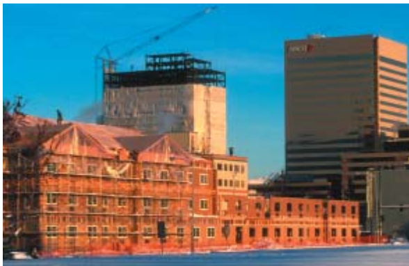
New hotel construction in downtown Anchorage
