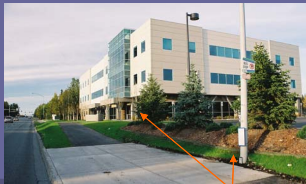
Transit accessible entrance
