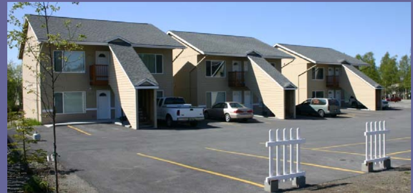
Existing conditions – landscaping and walkways
