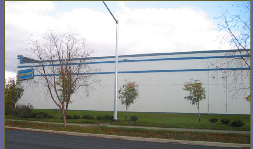
Existing Situation – Blank Wall Facing the Street
