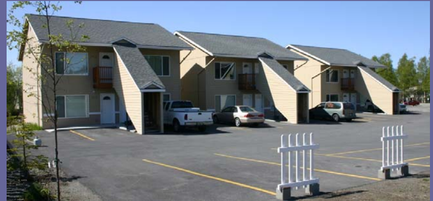
Existing conditions – landscaping and walkways
