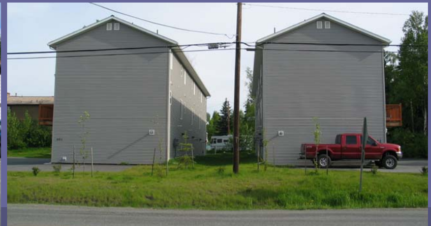
Existing conditions – blank walls
