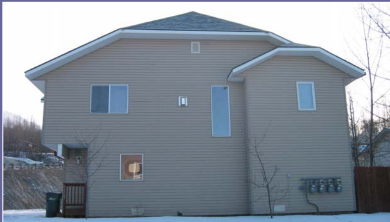
Street Facing End Façade
