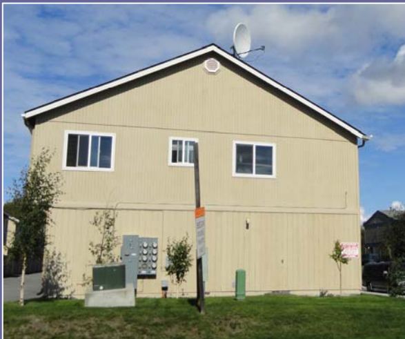
End Façade on side street
