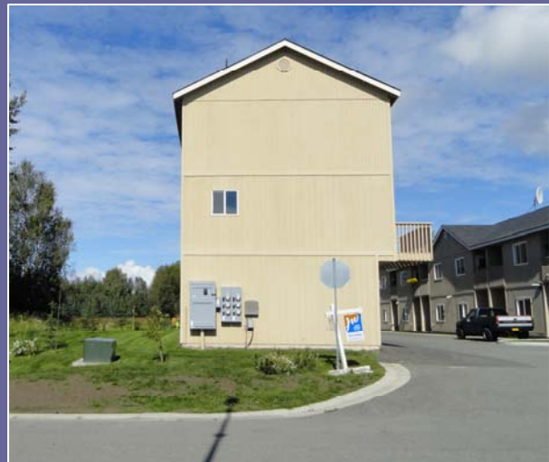
South Facing End Façade on Street
